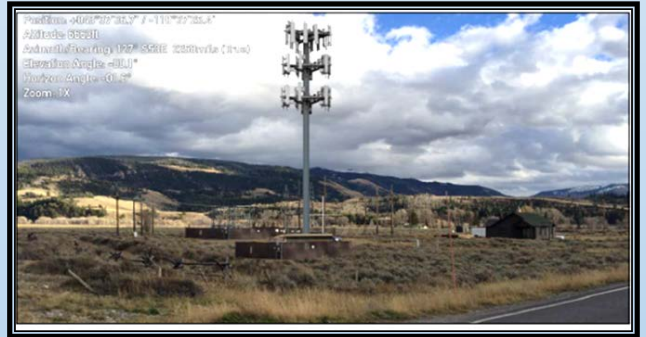
Original proposal at Kelly location with external antennas.
