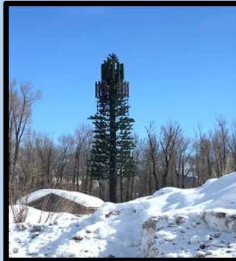
Examples of other types of camouflage poles from other locations.
