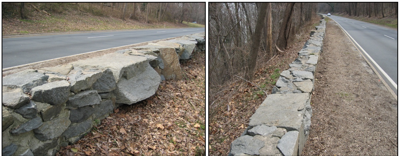
Figure 12. Photographs of Existing Stone Masonry Walls
