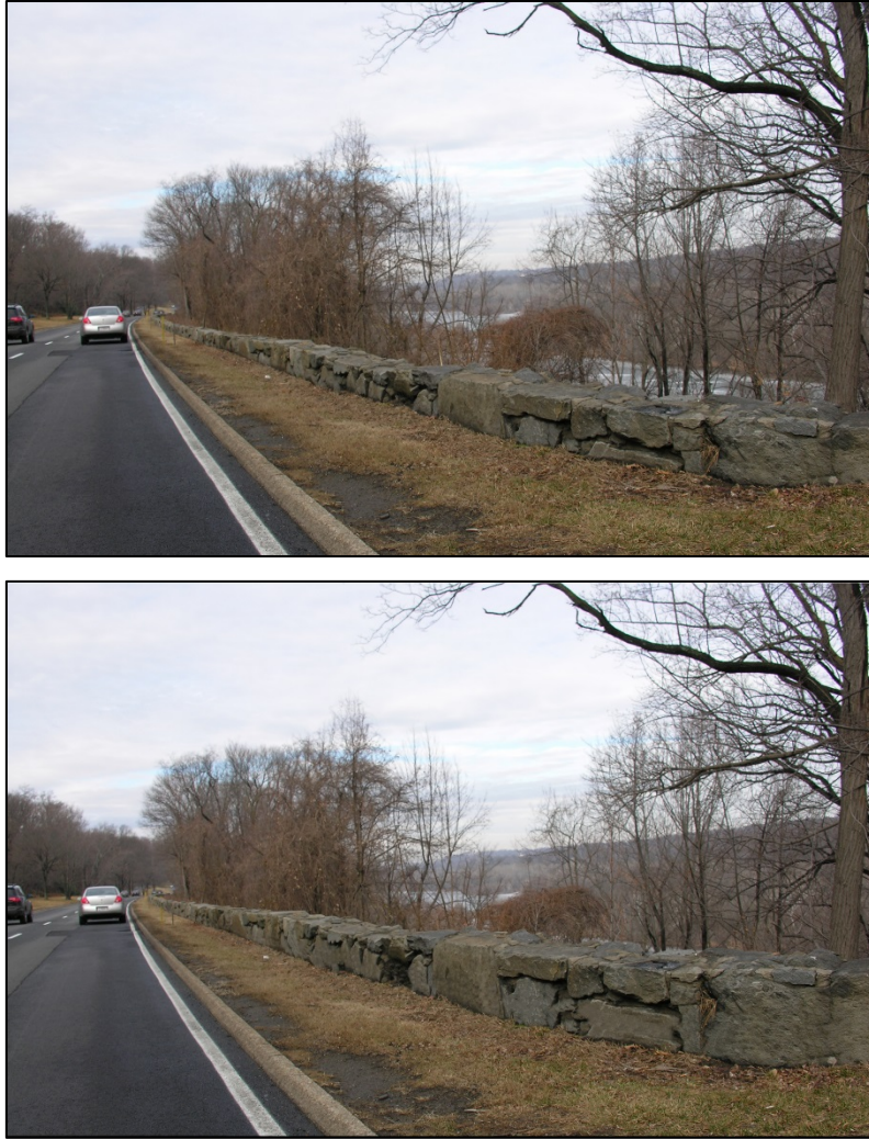
Figure 16. FHWA Design Visualization of Historic Stone Masonry Wall (top photo – existing wall; bottom photo – wall raised to 27 inches)
