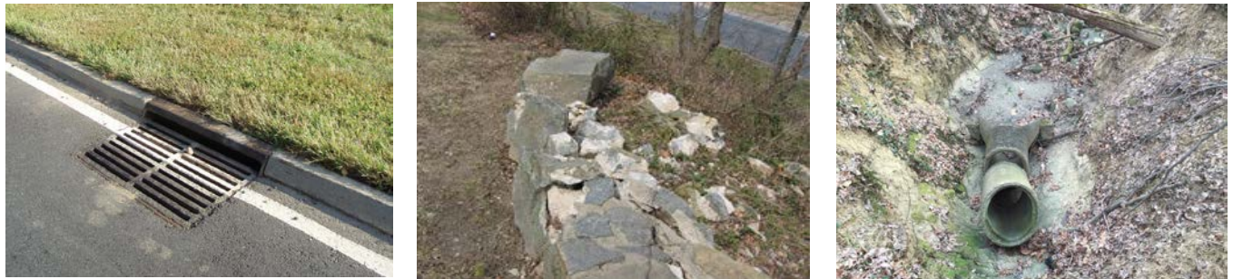
Figure 2. Examples of the project need (left photo – drop inlet in roadway, middle photo – stone wall in need of repair, and right photo – collapsed drainage pipe)
