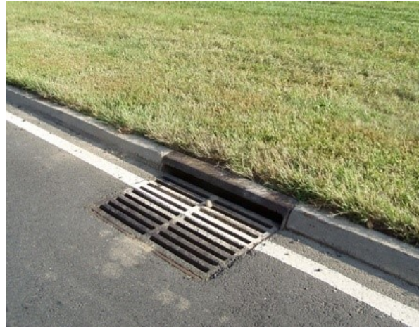
Figure 6. Current drainage grate inlet and curb opening
