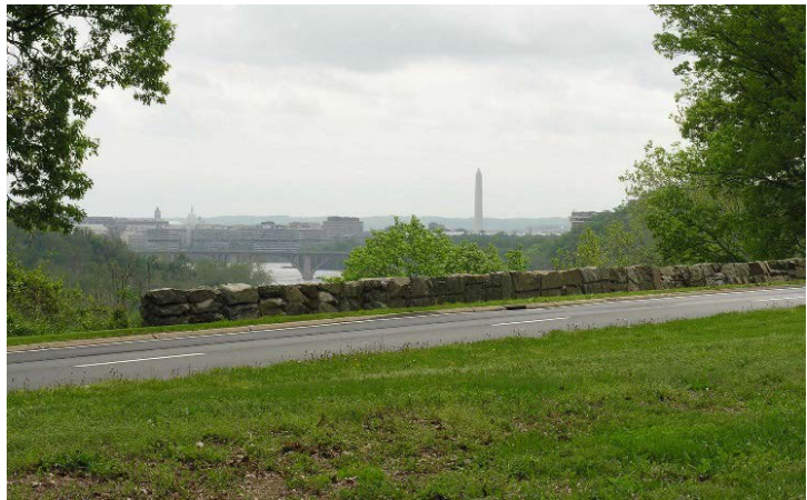
Figure 7. Photo rendering of 27-inch high stone masonry concrete-core guardwall
