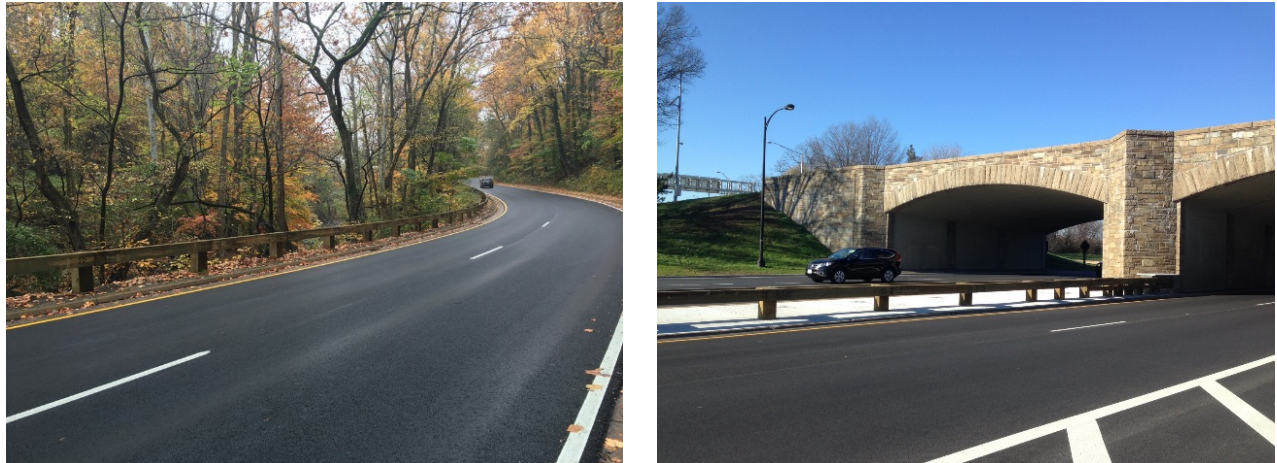
Figure 8. Two photos illustrating the placement of steel backed timber guardrail on the Parkway that would replace W-beam guardrails and Jersey barriers
