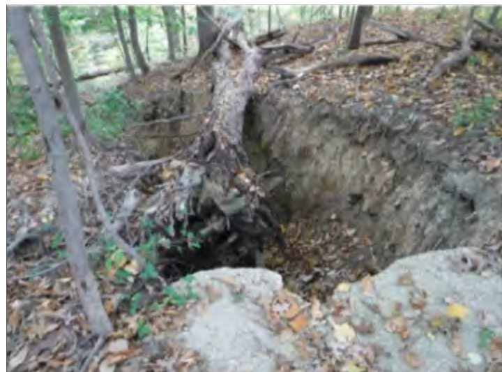
Example of erosion at outfall structure in need of repair and stabilization.
