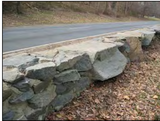
Figure 19. Defining wall character: The backside of an existing stone wall illustrates the multi-colored stones, varied sizes, depth and width of mortar
