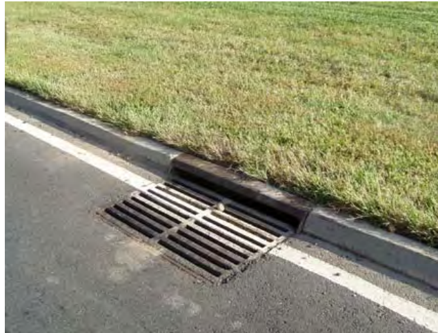
Figure 4. Current drainage grate inlet and curb opening
