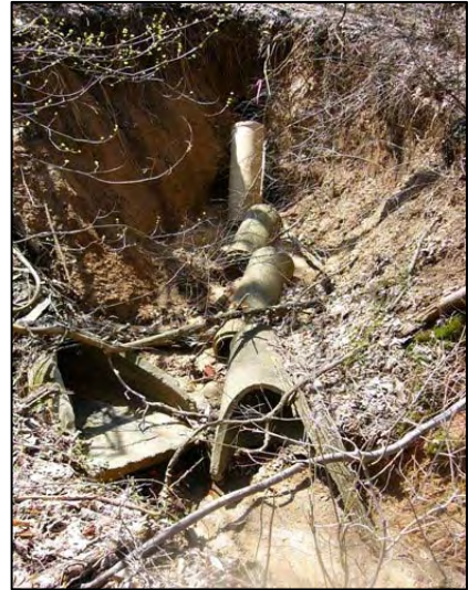
Figure 15. Undercutting at storm drain outfall
