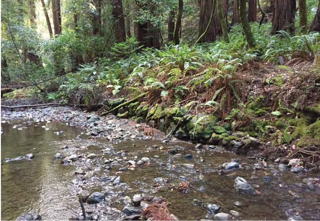
Figure 71. Overview, northwest stretch of Section R7, view south-southeast from creek bed, showing 2-3 courses of tightly stacked boulders of variable size with ferns and trees above
