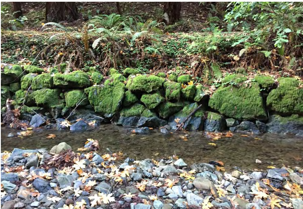
Figure 82. Detail, center-west stretch showing riprap in excellent condition with ferns above
