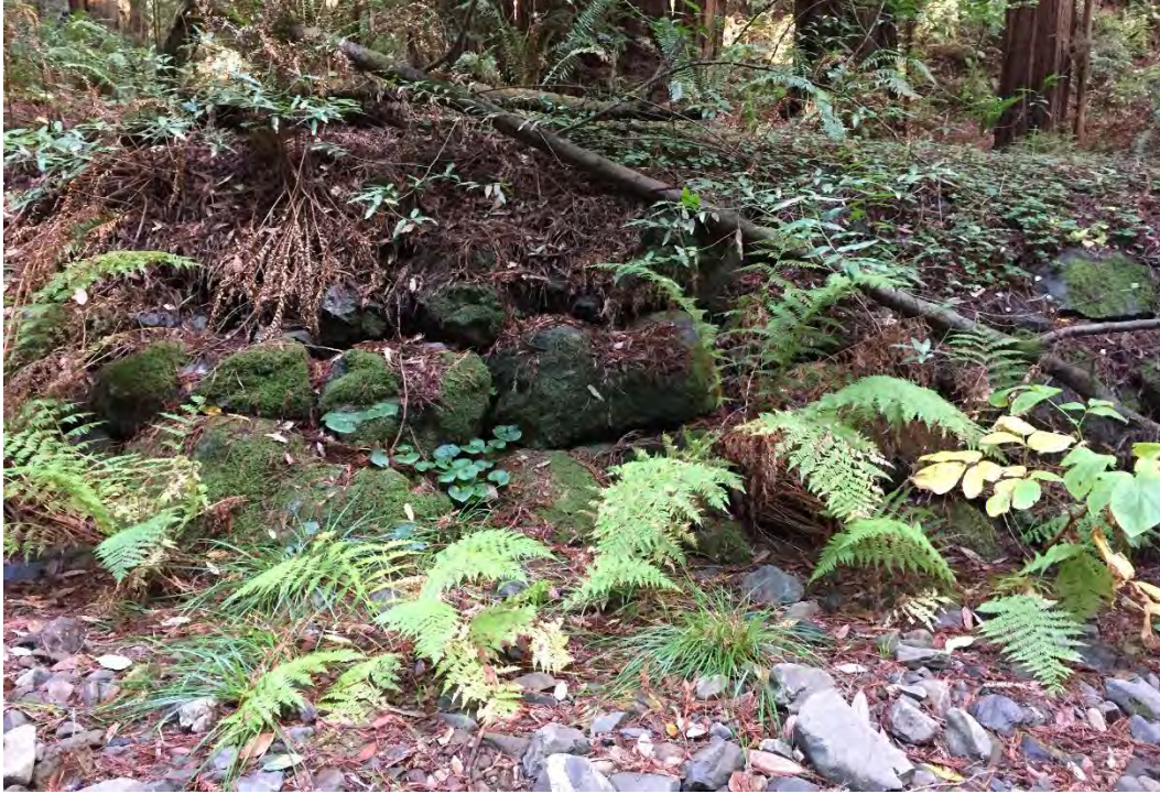
Figure 75. West stretch, view north from creek bed, showing riprap in fair condition beneath vegetation
