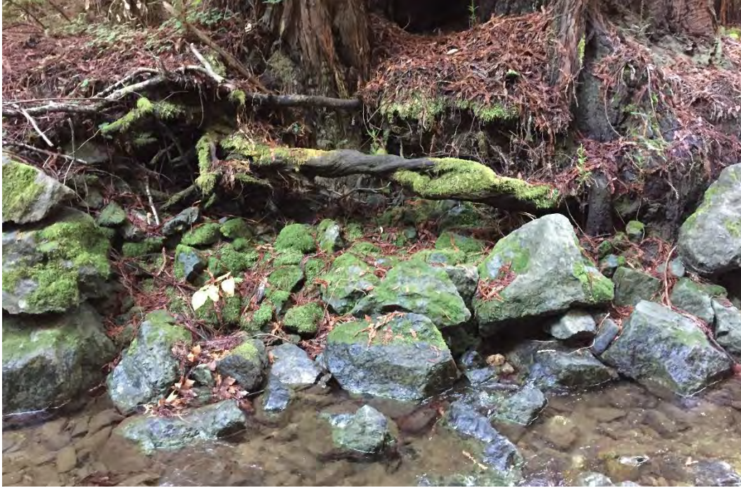
Figure 116. Central stretch showing large rocks pushed out by tree roots and smaller rocks used for backfill exposed
