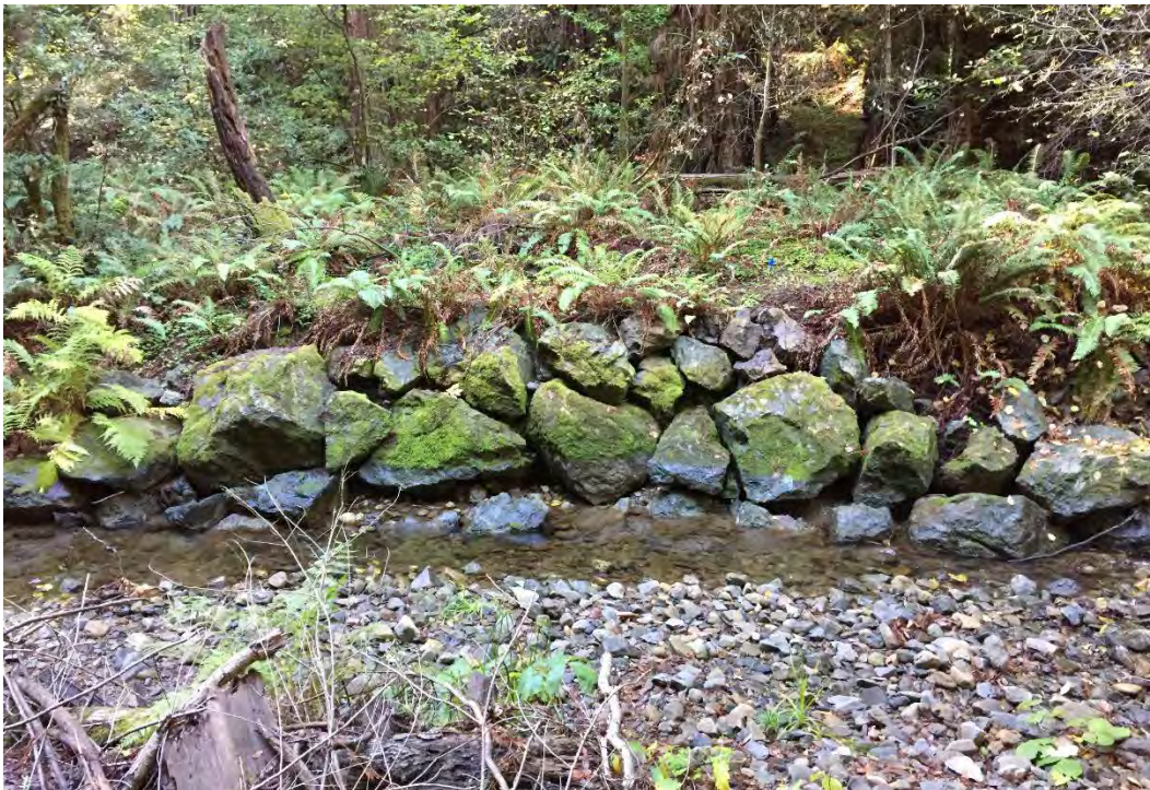
Figure 50. Center-south stretch of Section R6, view west-southwest showing riprap in clearly visible and in excellent condition with ferns above
