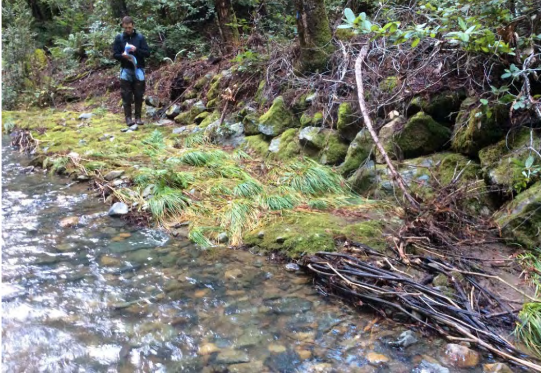
Figure 96. Upstream (west) stretch of Section L12 with toe material below riprap wall in good condition, view northeast from creek bed
