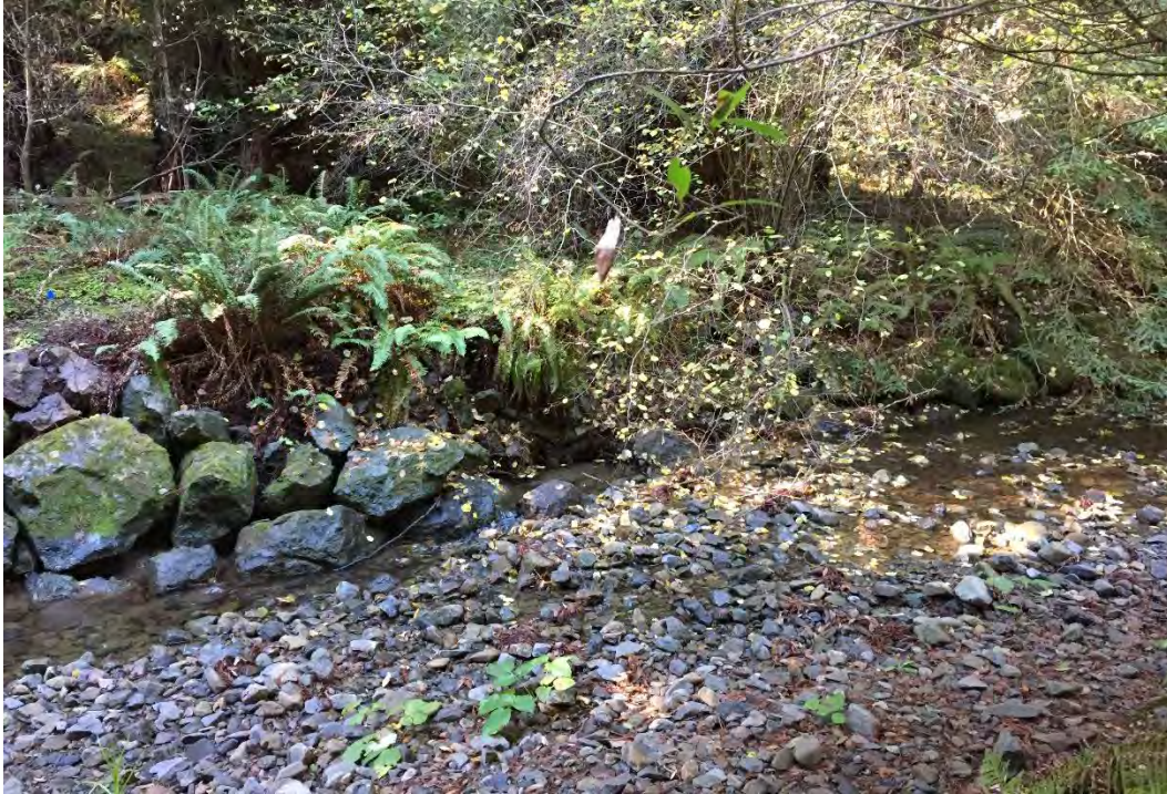
Figure 51. Center-north stretch of Section R6, showing riprap in good condition to south with area obscured by ferns and other vegetation to north
