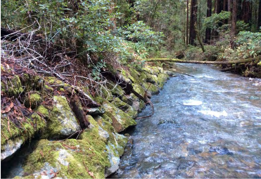
Figure 98. Downstream stretch of Section L12, view west from creek bed, showing riprap tightly-stacked and in excellent condition
