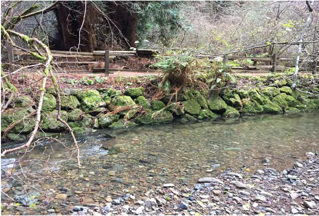
Figure 27. Section R3A from left bank with path visible in background, camera facing southwest, showing center-west stretch with 4-5 course riprap in excellent condition with minimal vegetation
