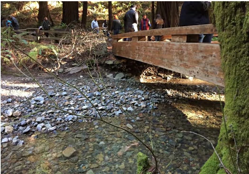
Figure 40. View of Section L4 from right bank, camera facing north, with little intact riprap in place
