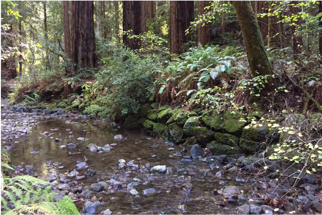
Figure 92. Overview of Section R9, view southeast from creek bed, showing riprap tightly stacked into 3 to 4 courses that form a nearly upright wall beneath trees, ferns, and other vegetation
