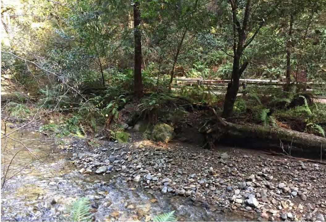
Figure 54. Section L6 from right bank, camera facing northeast, showing riprap in poor condition center frame and otherwise obscured by vegetation
