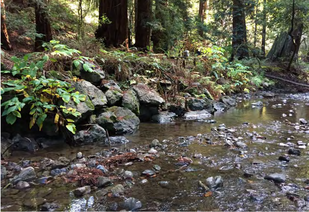
Figure 77. Center-east stretch, view east-northeast from creek bed, showing riprap in good condition
