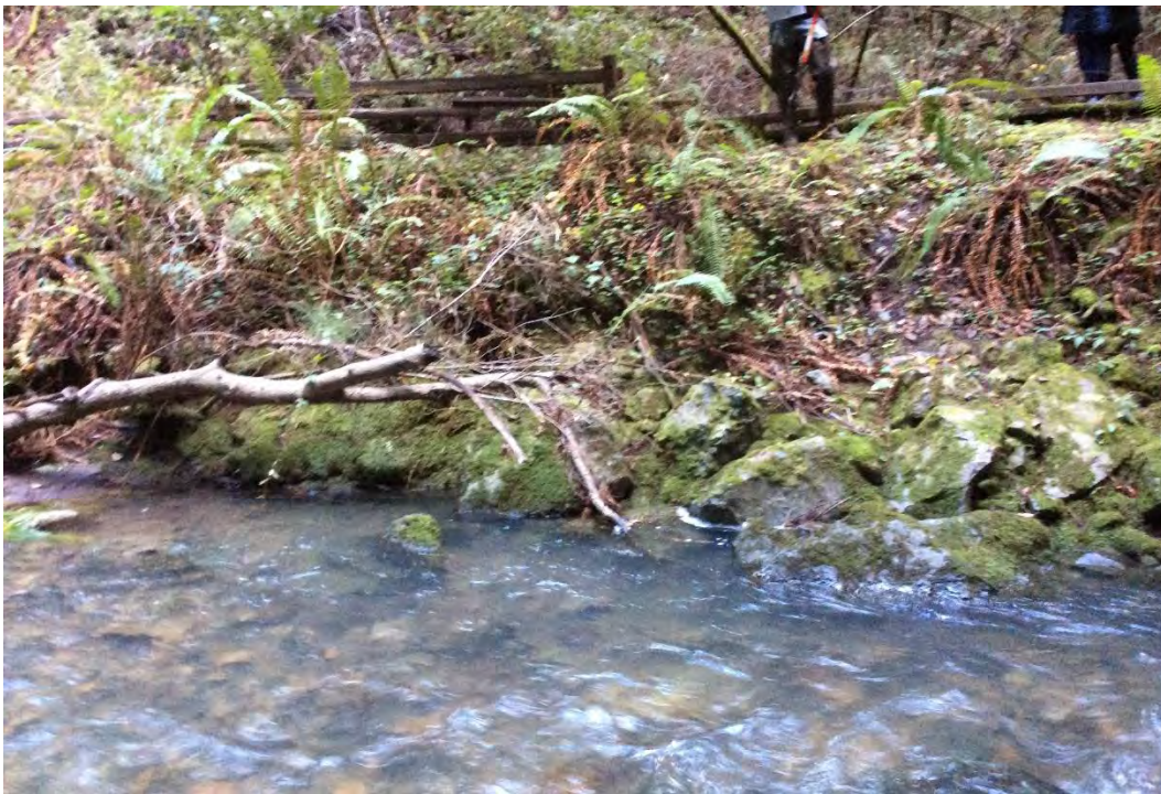
Figure 89. Center stretch of Section L11B, view northeast from creek bed, showing riprap in good condition with some woody debris and heavy moss growth
