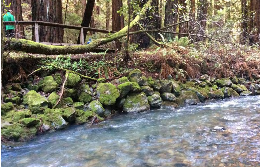
Figure 88. Downstream stretch of Section L11B looking east from creek bed, showing riprap in very good condition, with tightly stacked medium-sized rocks below fern growth
