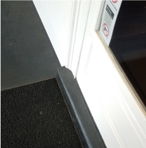
RAISED THRESHOLD AT ENTRANCE DOOR
