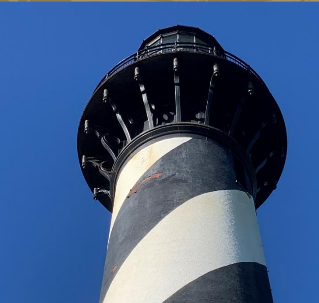
Exterior peeling paint
