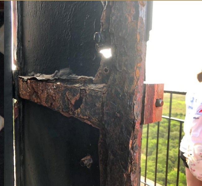
Corroded door
