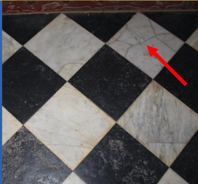
Broken floor tiles
