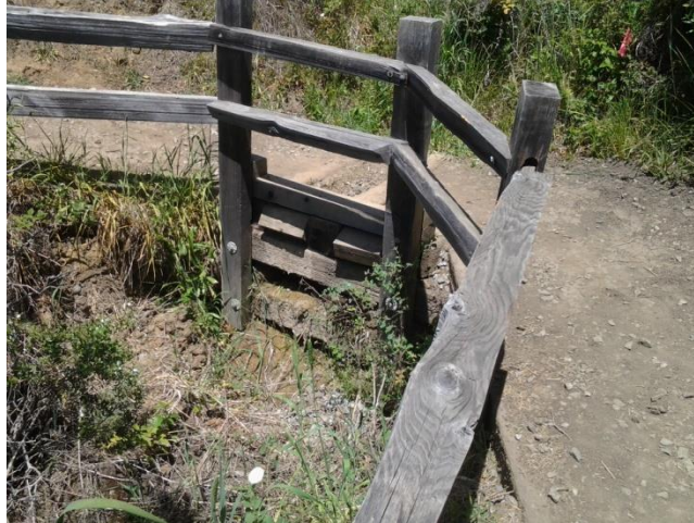
Figure 4. Crib wall at Bridge 11. Photo credit: GGNPC
