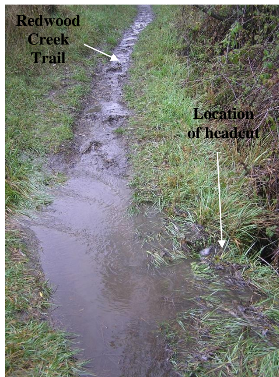
Figure 11. Erosion Site 1 is a small headcut that has developed immediately adjacent and downslope of Redwood Creek Trail (in the picture, the headcut is at bottom right where water is flowing off the trail). Photo credit: GGNPC
