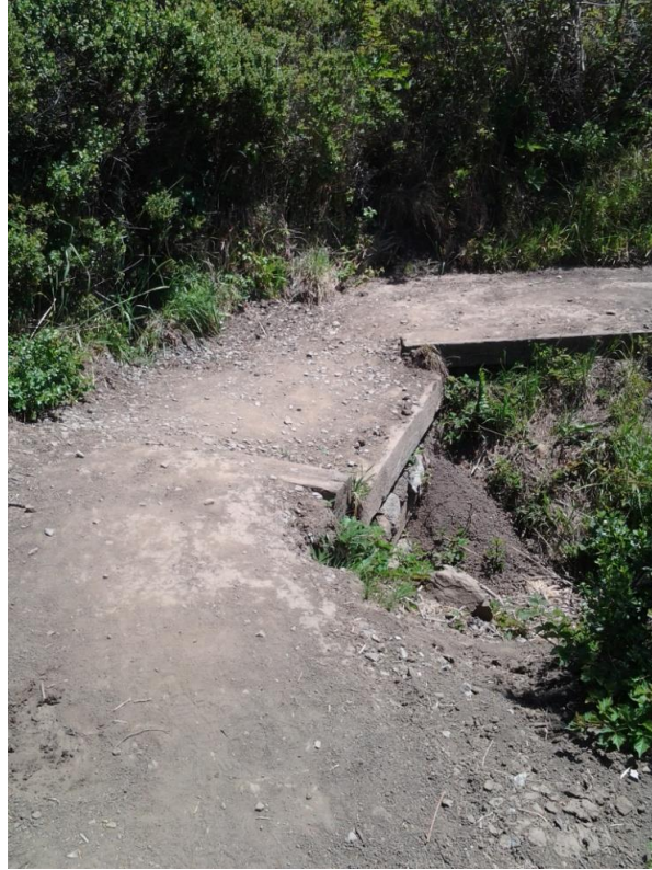
Figure 2. Crib wall at Bridge 10. Photo credit: GGNPC
