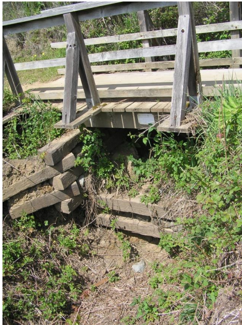
Figure 5. Crib wall at Bridge 12. A wood bridge spans the crib wall. Photo credit: GGNPC
