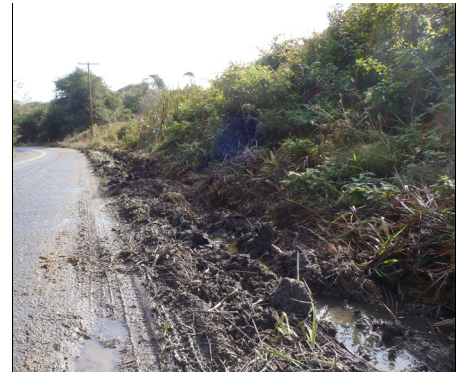
Large rut caused by vehicle running off the road in flood-prone area
