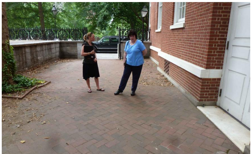
Photo 1: Kathryn (NPS) and Debby (Hunt Engineering) standing on area that is raised from tree root growth (note hump on tree pit border). This raised area is directing stormwater towards Library Hall entrance on right.
