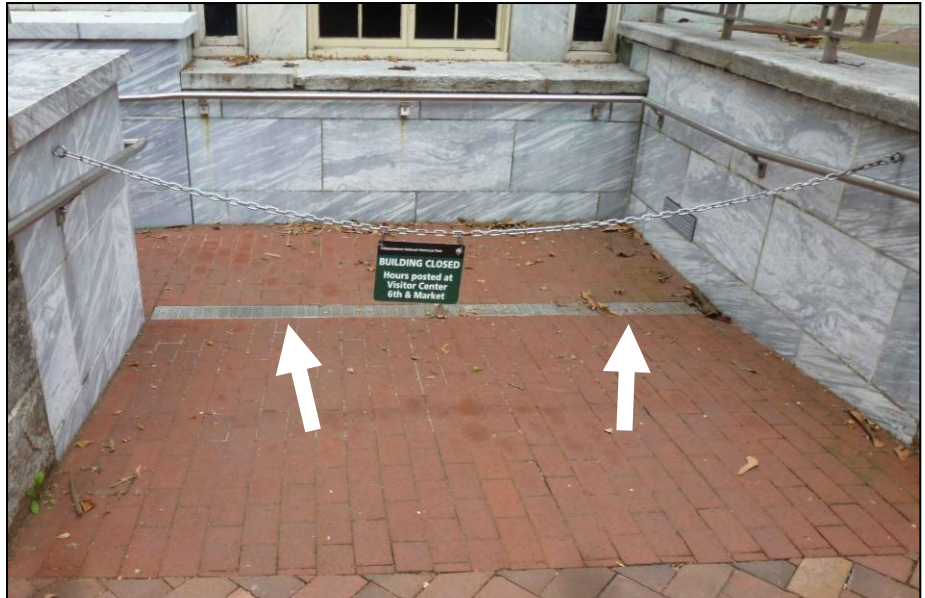
Photo 3: Trench drain on basement walkway
