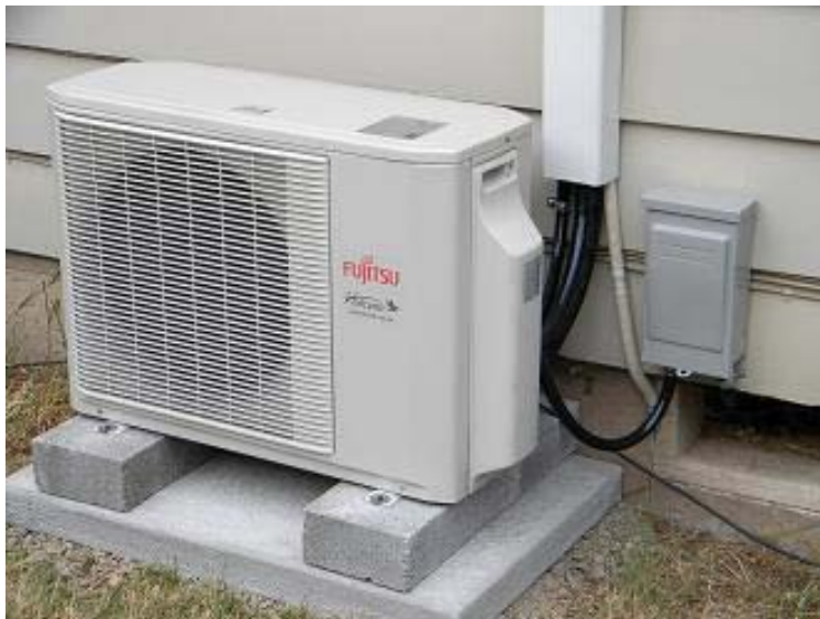
Ductless split-system heat pump unit of the type that would be installed outside the lodge.
