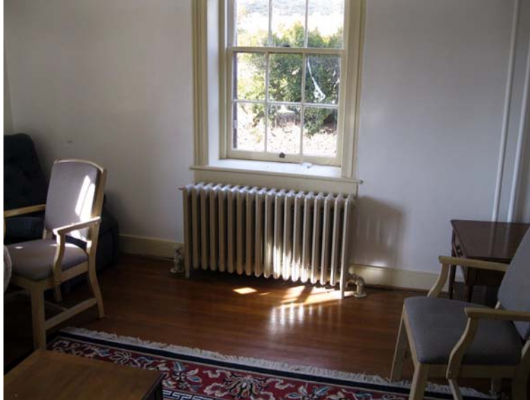
Typical radiator on the first floor. Radiators will be removed and replaced with ductless floor-mounted air handlers. Electrical and refrigerant lines will access the handlers through the existing floor holes that currently service the radiators.
