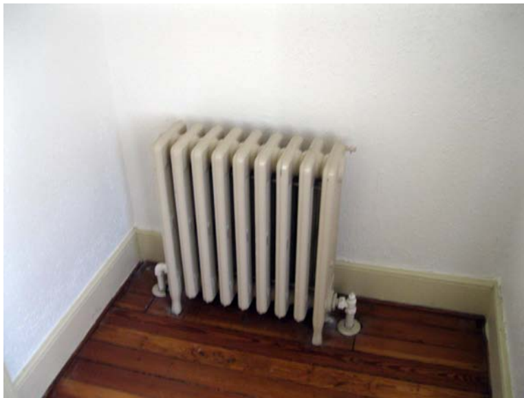
Typical radiator on the second floor. Radiators will be removed and replaced with ductless floor-mounted air handlers. Electrical and refrigerant lines will access the handlers through the existing floor holes that currently service the radiators.
