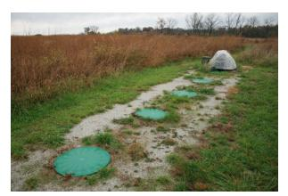
FIGURE 174. Above ground portions of the septic system. 17
