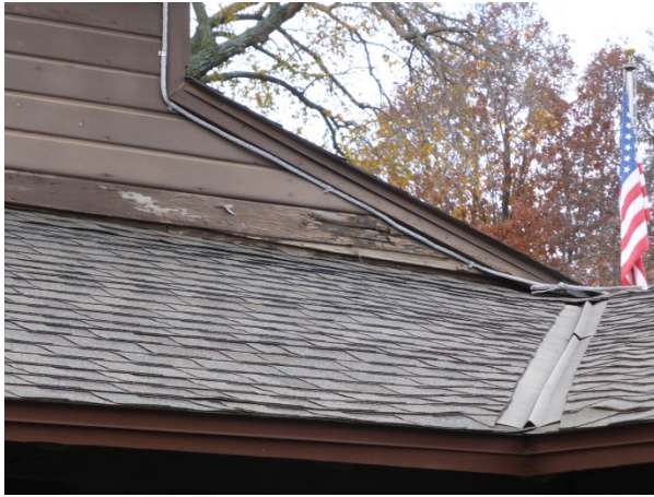
FIGURE 137. Detail showing the deteriorated siding and paint at the junction of the breezeway roof and the visitor center.
