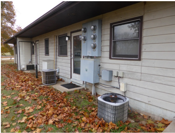
FIGURE 156. Detail of the rear of the building, showing stoops, condensing units, and electrical service features.
