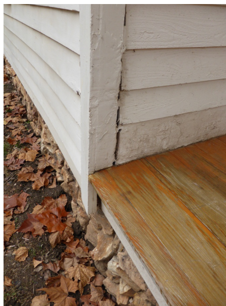
7 FIGURE 131. Detail of the junction of the front porch 8 and the main house showing the separation of siding 9 and porch elements caused by settlement and 10 movement.
