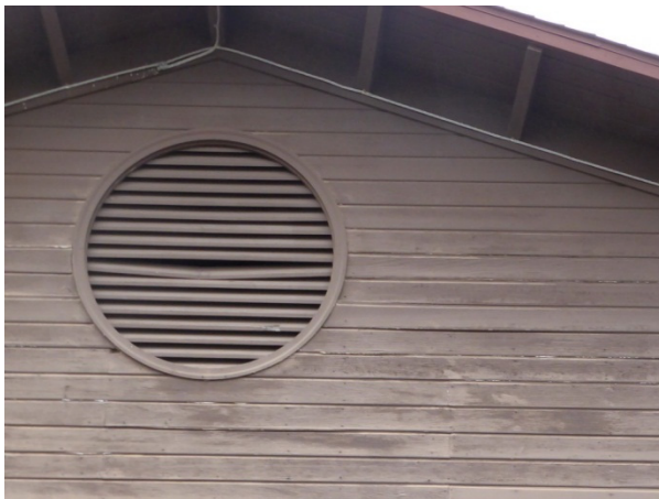
FIGURE 138. Detail of the warped and deteriorated wood siding and paint, as well as the damaged ridge vent, under the roof.
