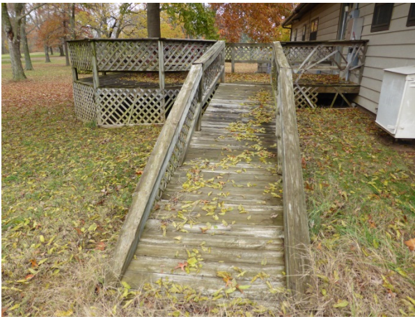
FIGURE 146. Detail of a deteriorated wood ramp and deck behind the Superintendent's residence.
