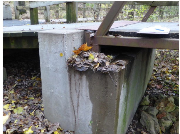
21 FIGURE 160. Detail of the concrete foundation stem 22 wall on Bridge 1.
