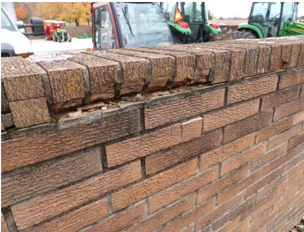
5 FIGURE 142. Detail of the deteriorated masonry wall 6 surrounding the maintenance yard.
