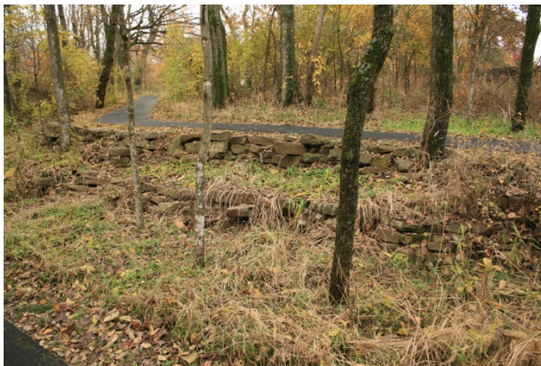
8 FIGURE 68. Low rock retaining walls and associated 9 grading were used to support the switchbacks.
