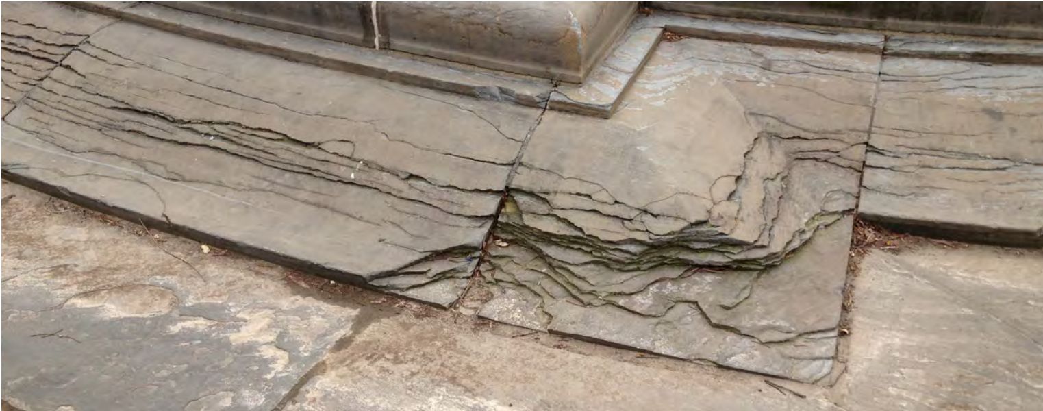
Spalling stone at the fountain
