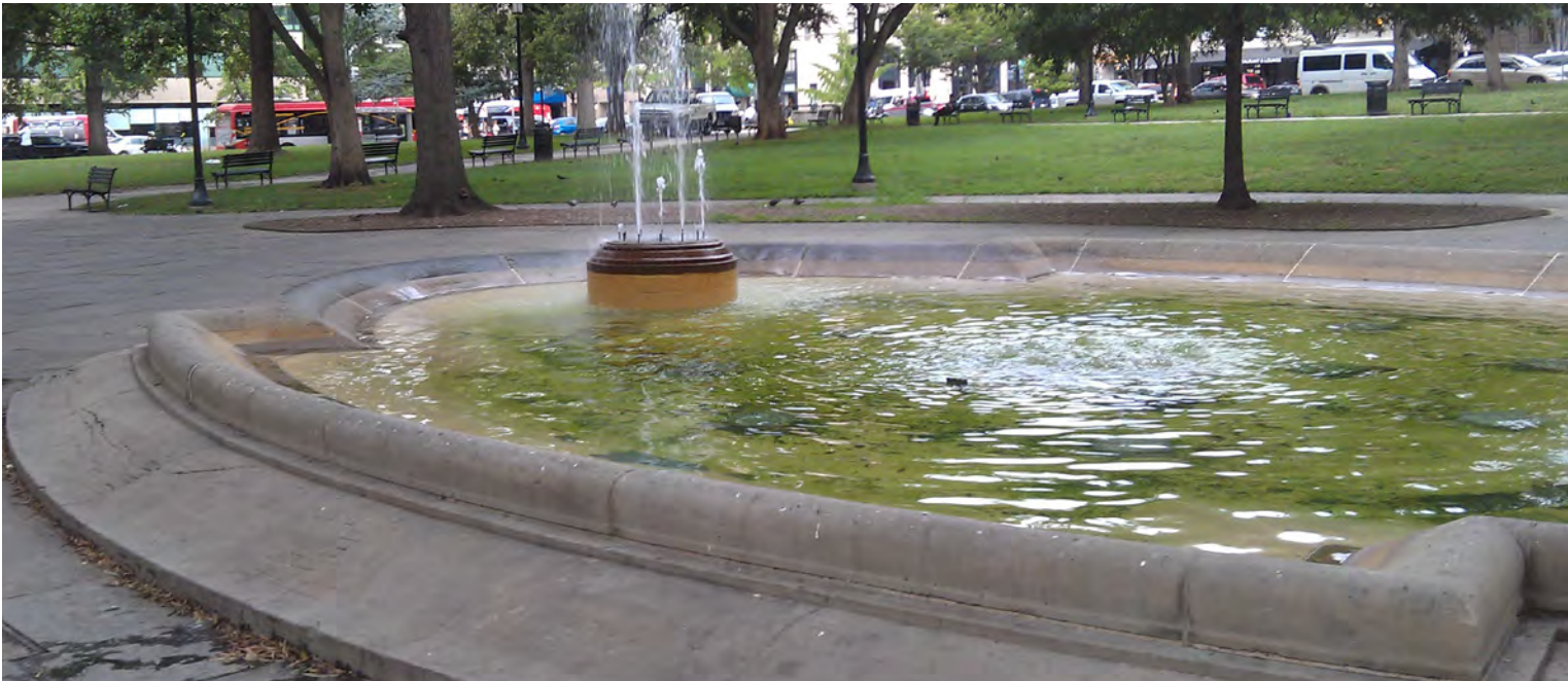
The fountain basin collects debris which settles at the bottom and algae bloom is frequent
