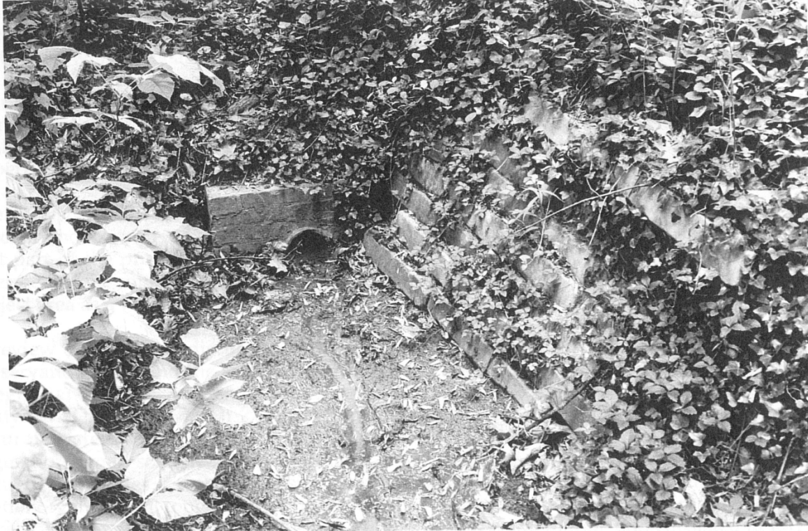
Figure 13 Brick Bulkhead with Headstone Embankment (Millis et al. 1998: 121)
