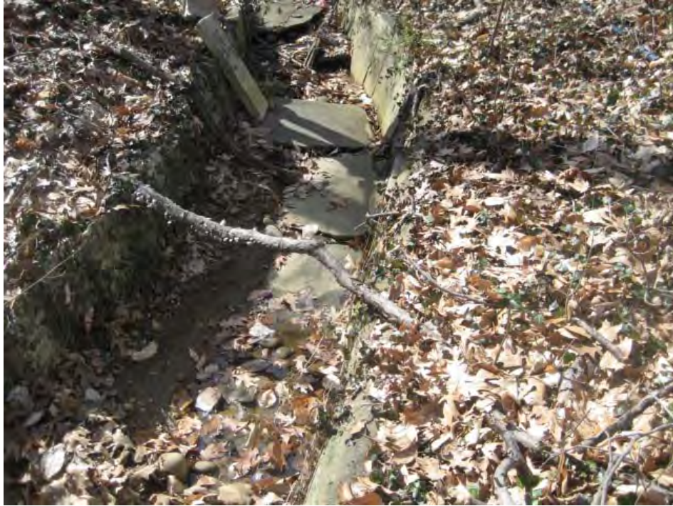
Figure 6 Upper Headstone Drain, Detail
