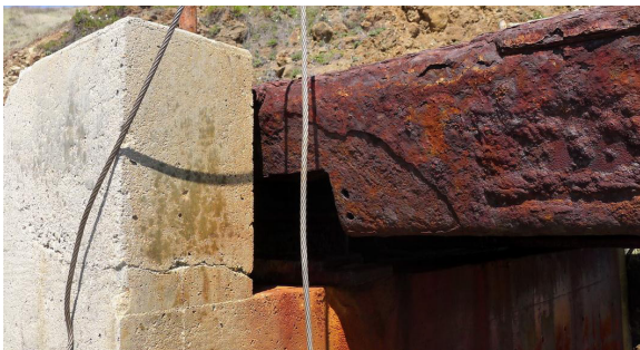
Photo 33. View of Scorpion Pier crack at concrete abutment wall.
