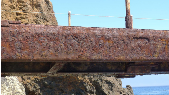
Photo 31. View of Scorpion Pier corroded exterior stringer at shore abutment.
