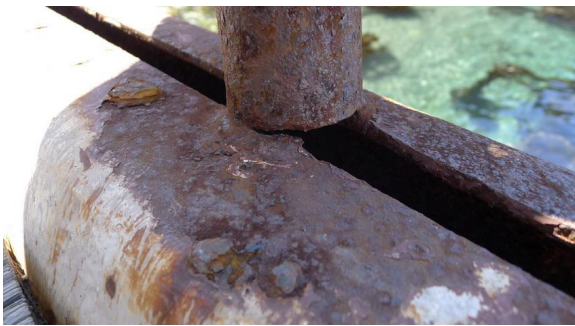
Photo 32. View of Scorpion Pier fractured weld connection at guardrail post base.
