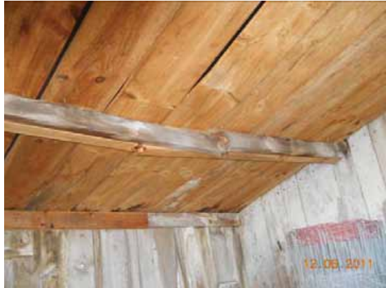
Figure 3-153: Cracked original and new 2x4 purlins, PD 12/6/11
