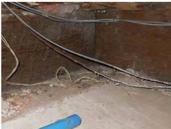
40 Figure 3-86: Embedded wood sill plate on the 41 stone foundation wall, northeast corner of the 42 basement, PD 12/6/11
