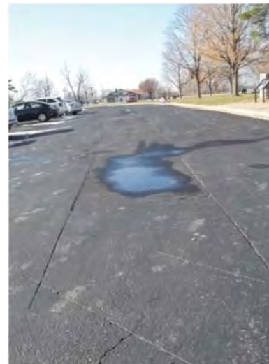
Figure 3-91: Patched asphalt where geothermal wells installed in parking lot, DMD 12/6/11
