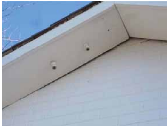
Figure 3-142: Garage Building Knob and Tube Connectors, Jon Brooks 12/6/11
