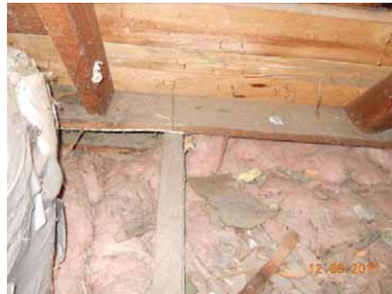
Figure 3-87: West wing attic, rafters do not align with ceiling joists, PD 12/6/11
