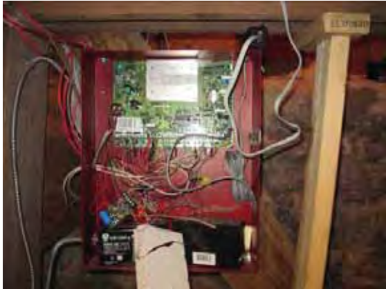
Figure 3-114: Existing security and fire alarm control panel, Jon Brooks 12/6/11
