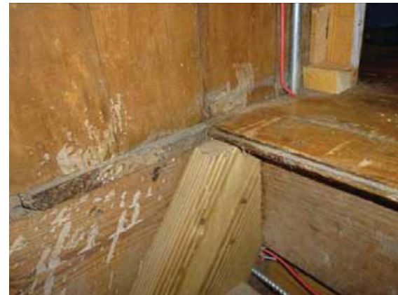
Figure 3-82: Central wing tongue and groove floor, as seen from the basement stair, ABA 12/6/11
