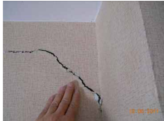
Figure 3-122: West wing wall cracking, second floor hall 201 adjacent to north chimney, PD 12/6/11
