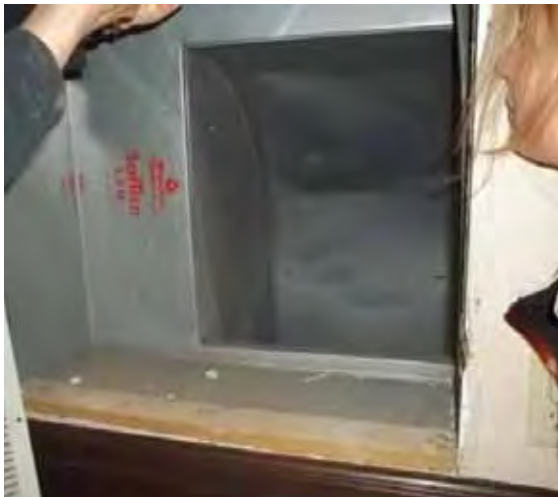
Figure 3-97: Ductwork behind return air grille, DMD 12/6/11
