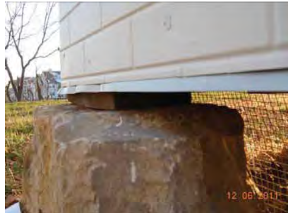
Figure 3-141: Stone supporting Garage corner, PD 12/6/11
