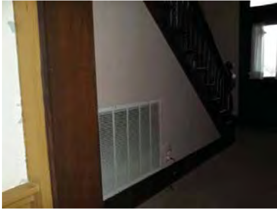
Figure 3-96: Return air grille below stairs, DMD 12/6/11
