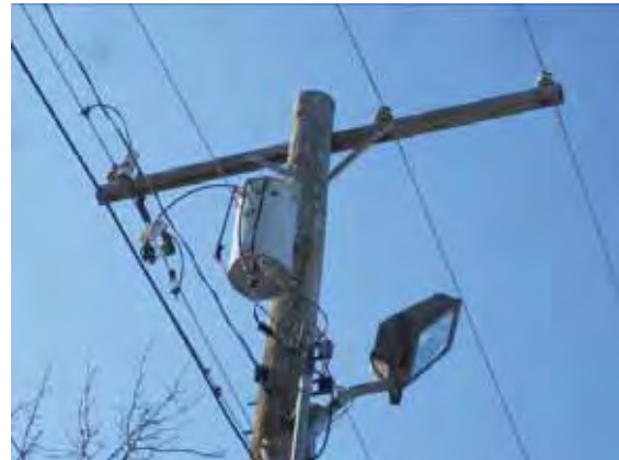
Figure 3-108: Existing pole mounted transformer, Jon Brooks 12/6/11
