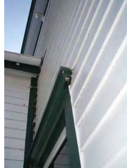
Figure 3-118: Separation of central and east wing, EMH 12/6/11
