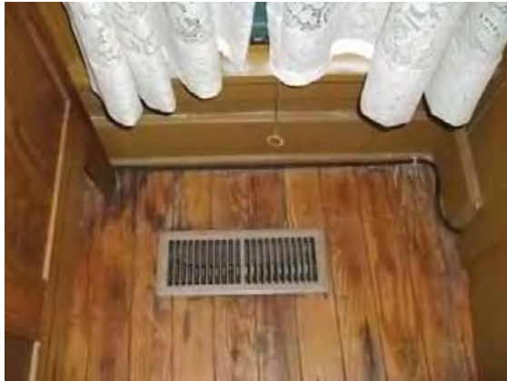
18 Figure 3-92: Typical floor diffuser, DMD 12/6/11
