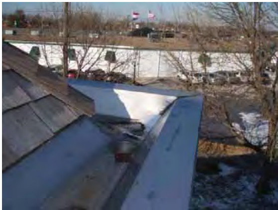
Figure 3-117: c.1984 stainless steel integral gutter, minor damage at corner joint, EMH 12/6/11
