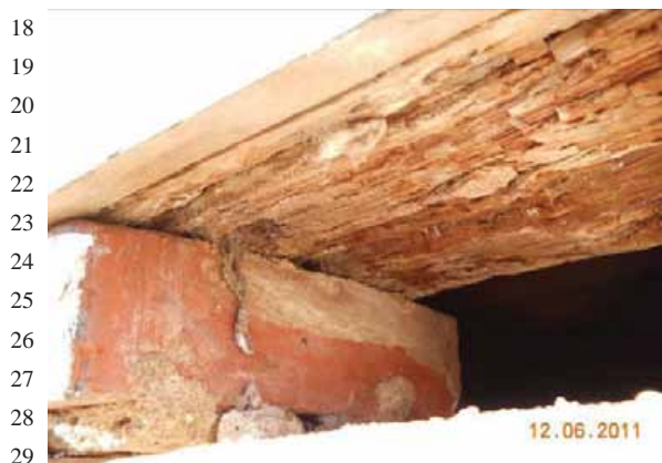
Figure 3-126: Decayed wood sill plate (or beam?) on brick grade beam, south wall west wing, PD 12/6/11
