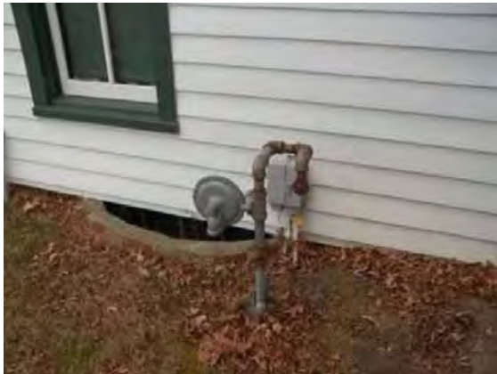
Figure 3-107: Gas line stubbed up with pressure regulator and no meter, DMD 12/6/11
