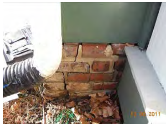
Figure 3-124: Deteriorated bricks and mortar, brick grade beam, southeast corner of west wing, PD 12/6/11
