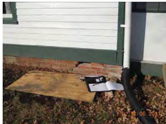
Figure 3-125: Cracking and Rowlock brick easily removed from south grade beam of west wing, PD 12/6/11
