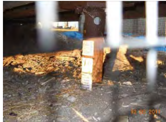
Figure 3-139: Helical pile, PD 12/6/11
