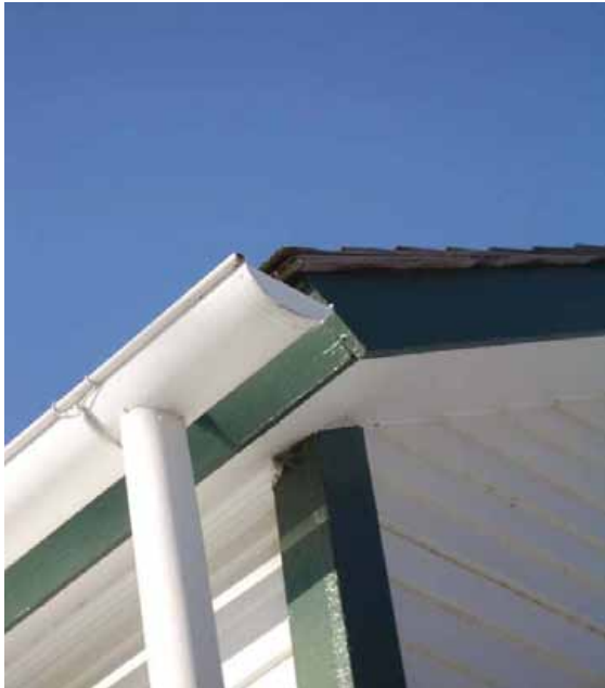
Figure 3-57: Half round gutter and round downspout, EMH 12/6/11
