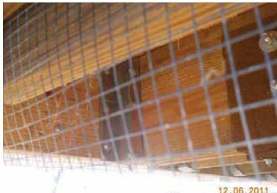
Figure 3-140: Angle connecting rim joist to built-up beam, PD 12/6/11
