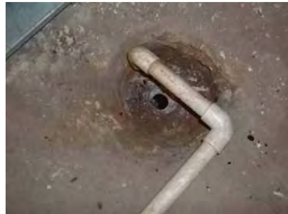
Figure 3-106: Floor drain in basement, DMD 12/6/11
