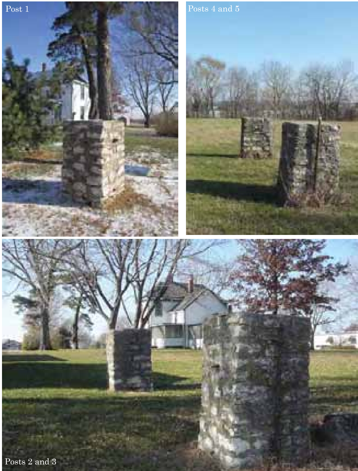
1 Figure 3-22. There are five standing stone posts built of coursed limestone and mortar with concrete 2 caps. The posts occur along an east west line south of the Farm Home and historically supported 3 fences and gates. SS 12/6/11; BN 11/23/11
