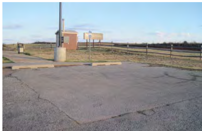
Poor pavement condition in parking lot at Washita Battlefield. Source: National Park Service
