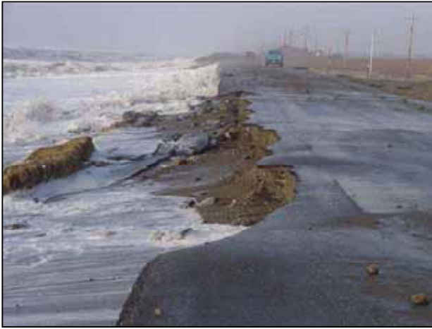
Coastal Erosion on Nome Council Road (ADOT&PF)
