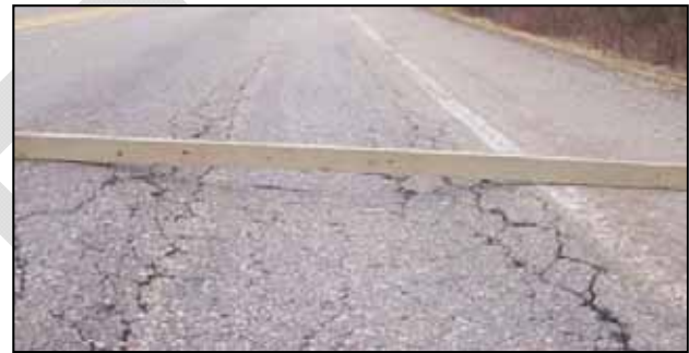
Elliott Highway, Pavement Rutting
