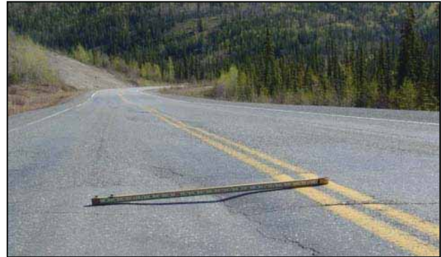
Alaska Highway, Damage and Rutting
