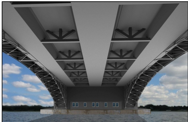
Figure 14: Conceptual rendering of the concrete box girder replacement structure proposed under Alternative 1A (Underside View)
