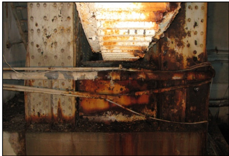
Figure 11: View of severe corrosion of the inner trunnion post of the bascule span
