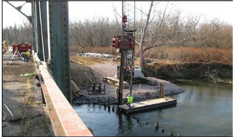
Figure 24: Example of Temporary Construction Causeway When construction activities are complete, the causeways would be removed and the river bottom restored to its current condition. Figure 24 provides an example of a temporary construction causeway.
