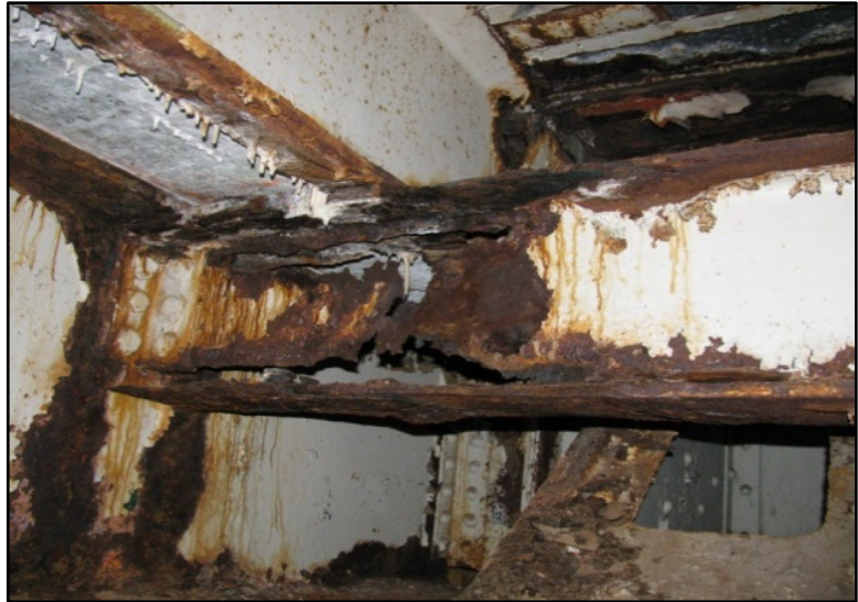
Figure 63: Example of steel truss under sidewalk with severe corrosion that may require replacement
