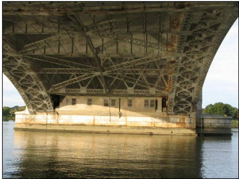
Figure 62: Steel truss bascule span that would be rehabilitated in place under Alternative 3
