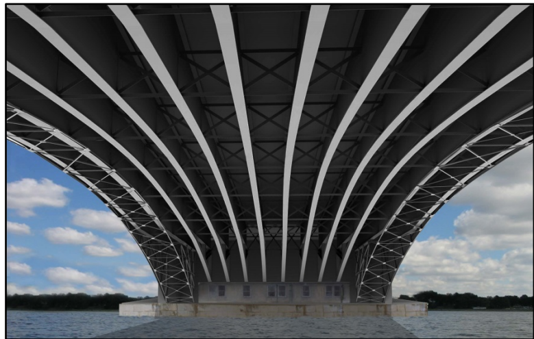
Figure 16: Conceptual rendering of the variable depth steel girder replacement structure proposed under Alternative 1B (Underside View)
