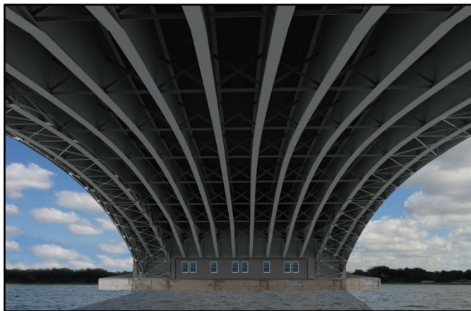
Figure 60: Conceptual rendering of the variable depth steel girder replacement structure proposed under Alternative 1B (Underside View)
