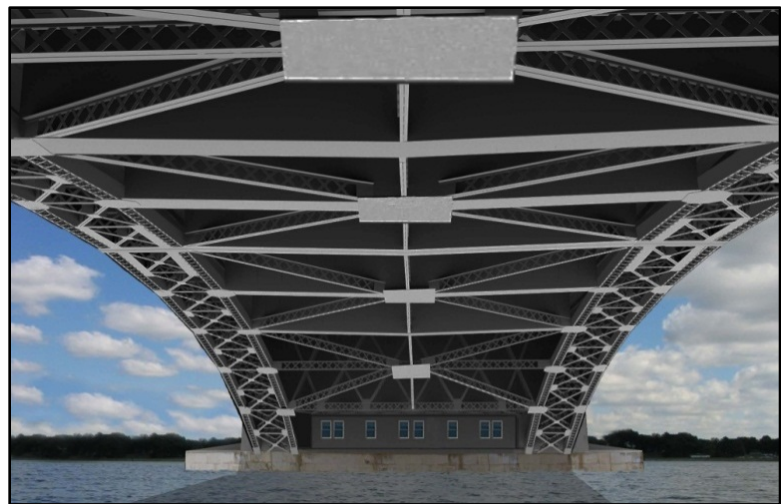
Figure 17: Conceptual rendering of the welded steel truss replacement structure proposed under Alternative 2 (Underside View)
