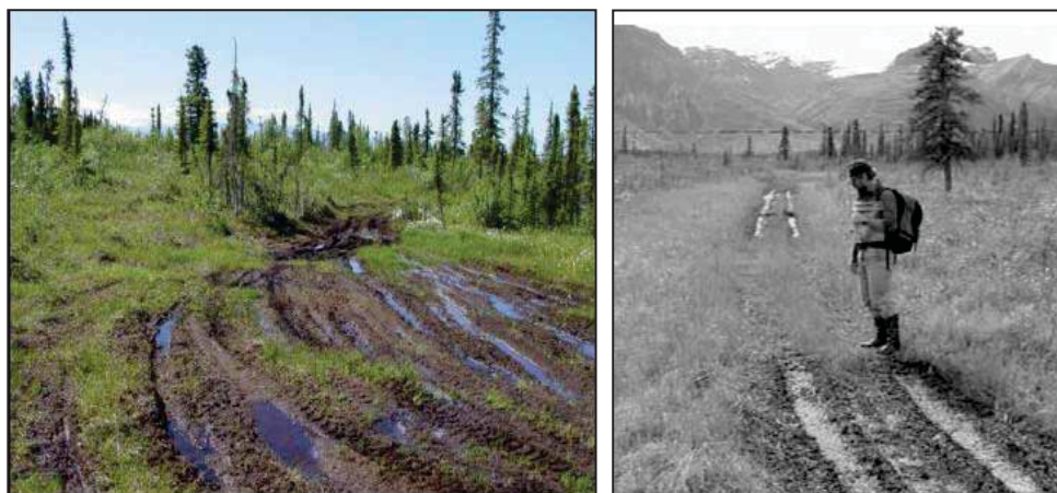
(left) - An example of ORV use in without hardened trail technology (NPS 2010). (right) - An experimental 40 foot section of hardened trail constructed with GeoBlock brand geogrid five years after installation (FHWA 2000).
