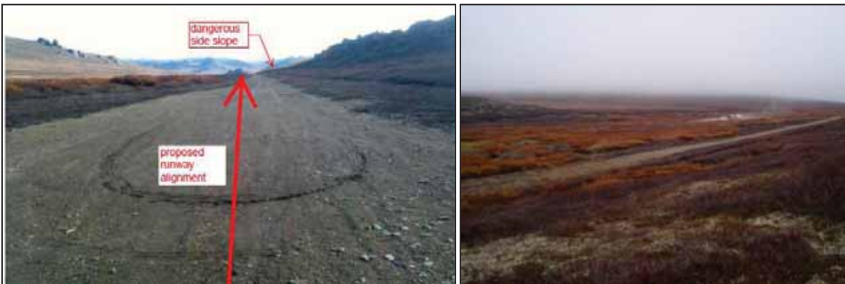
(left) - View of Serpentine Hot Springs airstrip looking southeast. The proposed alignment of the 1,500-foot airstrip would rotate the southeast 40 feet to avoid the side-slope on the right side of the airstrip (Crews, Oct 2010). (right) - Clearing vegetation at each end of the airstrip could lengthen the usable airstrip (Crews, Oct 2010).
