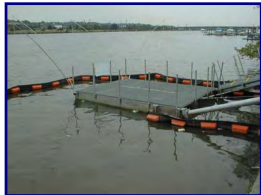
Floating End-Of-Pipe Netting System at CSO 018 – Anacostia River
