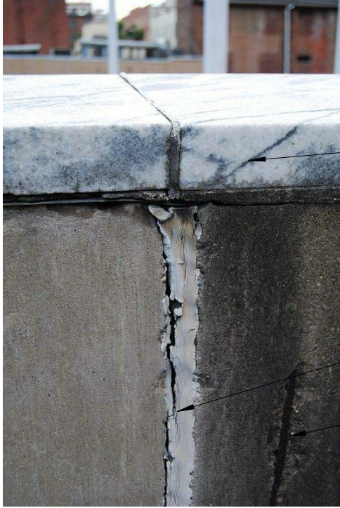
N. CONTROL JOINT AT BACK SIDE OF PARAPET WALL
