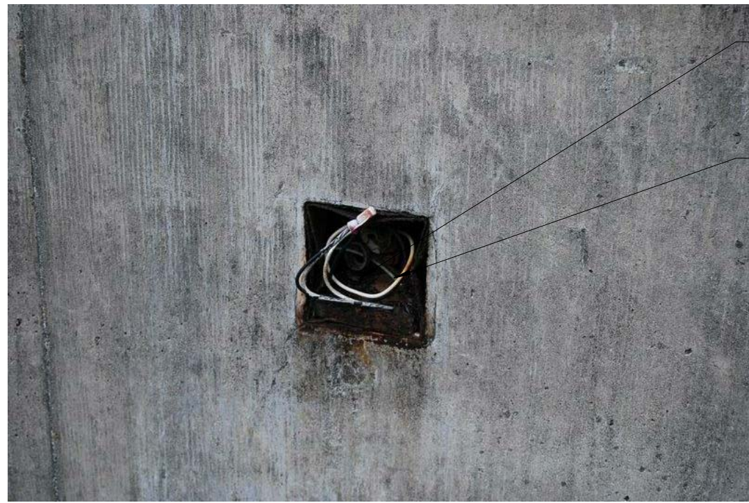
I. LIGHTING JUNCTION BOX AT BACK SIDE OF PARAPET WALL
