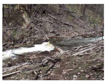
**Figure G-5.** Fish barrier constructed mostly of logs and rocks in 2008 to temporarily isolate East Fork Specimen Creek for restoration of native westslope cutthroat trout. Vegetation is recovering following the Owl Fire, which burned the watershed (including the barrier site) in 2007.
