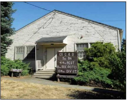
Figure 15. The west facade of building 728, showing distressed paint as one example of maintenance activities needed to stabilize and protect buildings in the East and South Barracks. (National Park Service)
