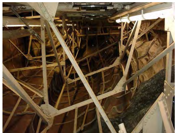
Figure 3.6 – View of Historic Structural Framework Inside statue
