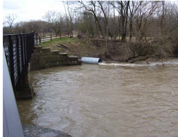
Figure 12. Outflow structure draining high water from canal into Tinkers Creek (April 2009)
