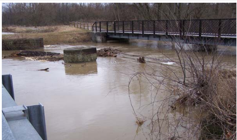
Figure 3. High water over existing steel pipes (March 9, 2009)
