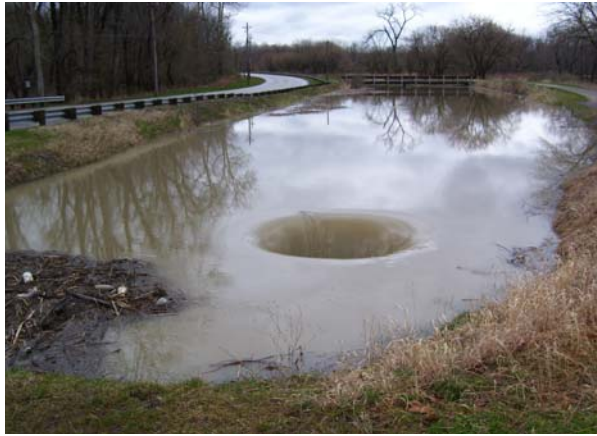
Figure 11. Riser in canal south of aqueduct draining high water (April 2009)
