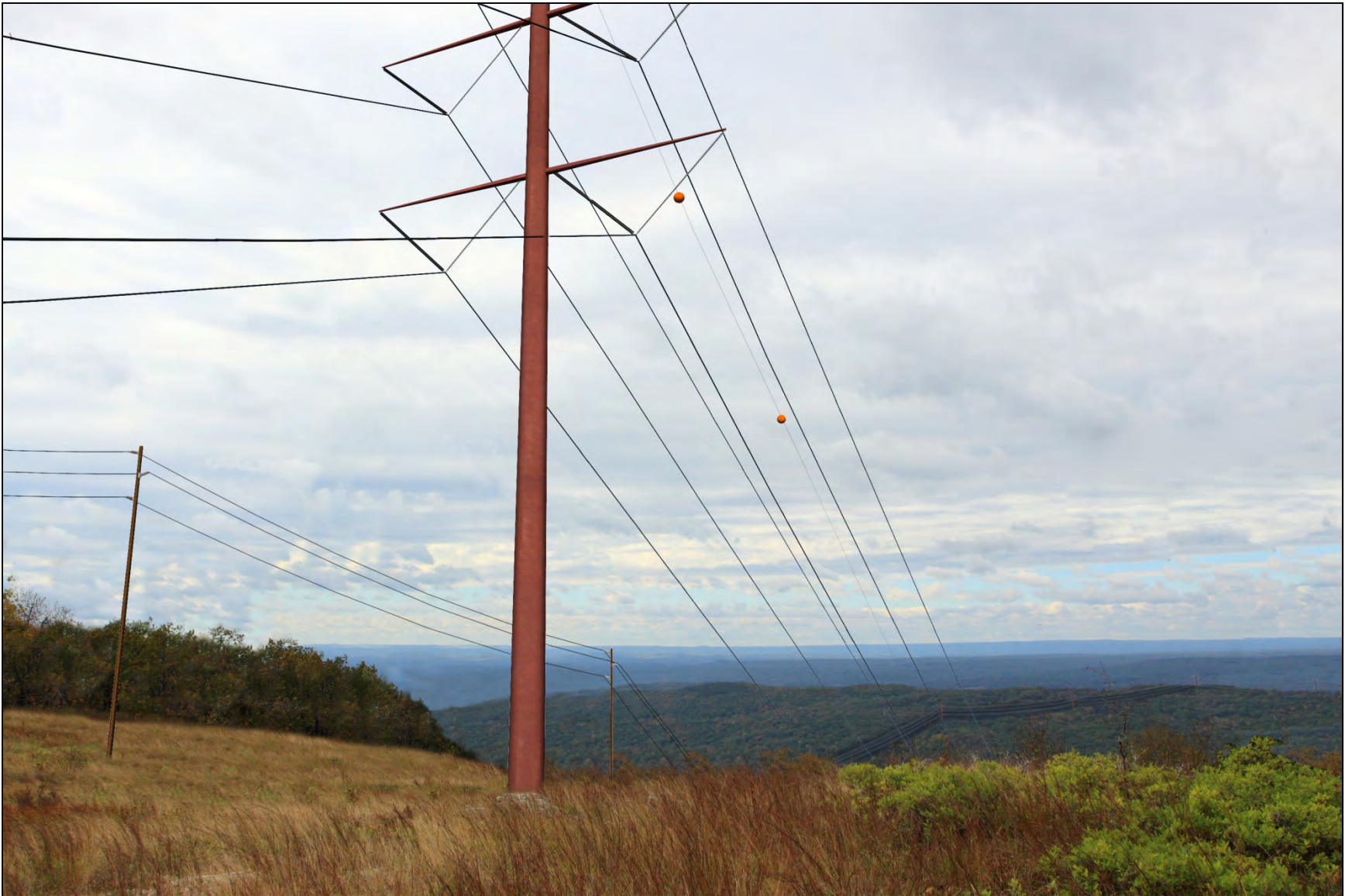
FIGURE 3-13B, PROPOSED: REPRESENTATIVE OF MIGRATORY BIRD DIVERter DEVICES (MARKER BALLS) ON THE STATIC WIRE. APLIC-APPROVED BIRD DIVERter DEVICES OF SOME TYPE WOULD BE REQUIRED WHERE ANY ALTERNATIVE ALIGNMENT CROSSES MDSR AND KITTATINNY RIDGE.
