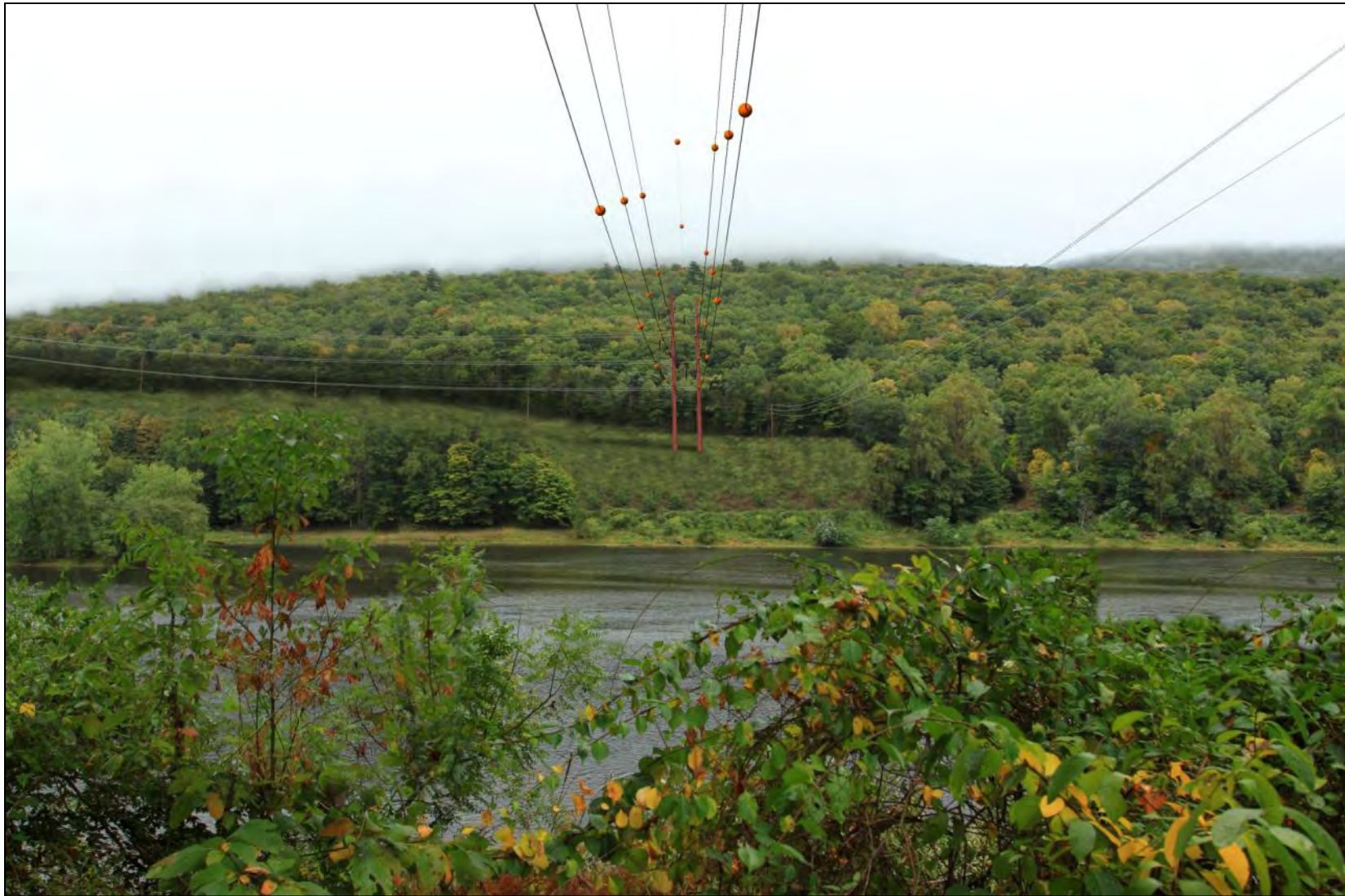
FIGURE 3-4B, PROPOSED. REPRESENTATIVE OF MIGRATORY BIRD DIVERTER DEVICES (MARKER BALLS) ON THE 500-kV CONDUCTORS. APLIC-APPROVED BIRD DIVERTER DEVICES OF SOME TYPE WOULD BE REQUIRED WHERE AN ALIGNMENT CROSSES MDSR AND KITTATINNY RIDGE.
