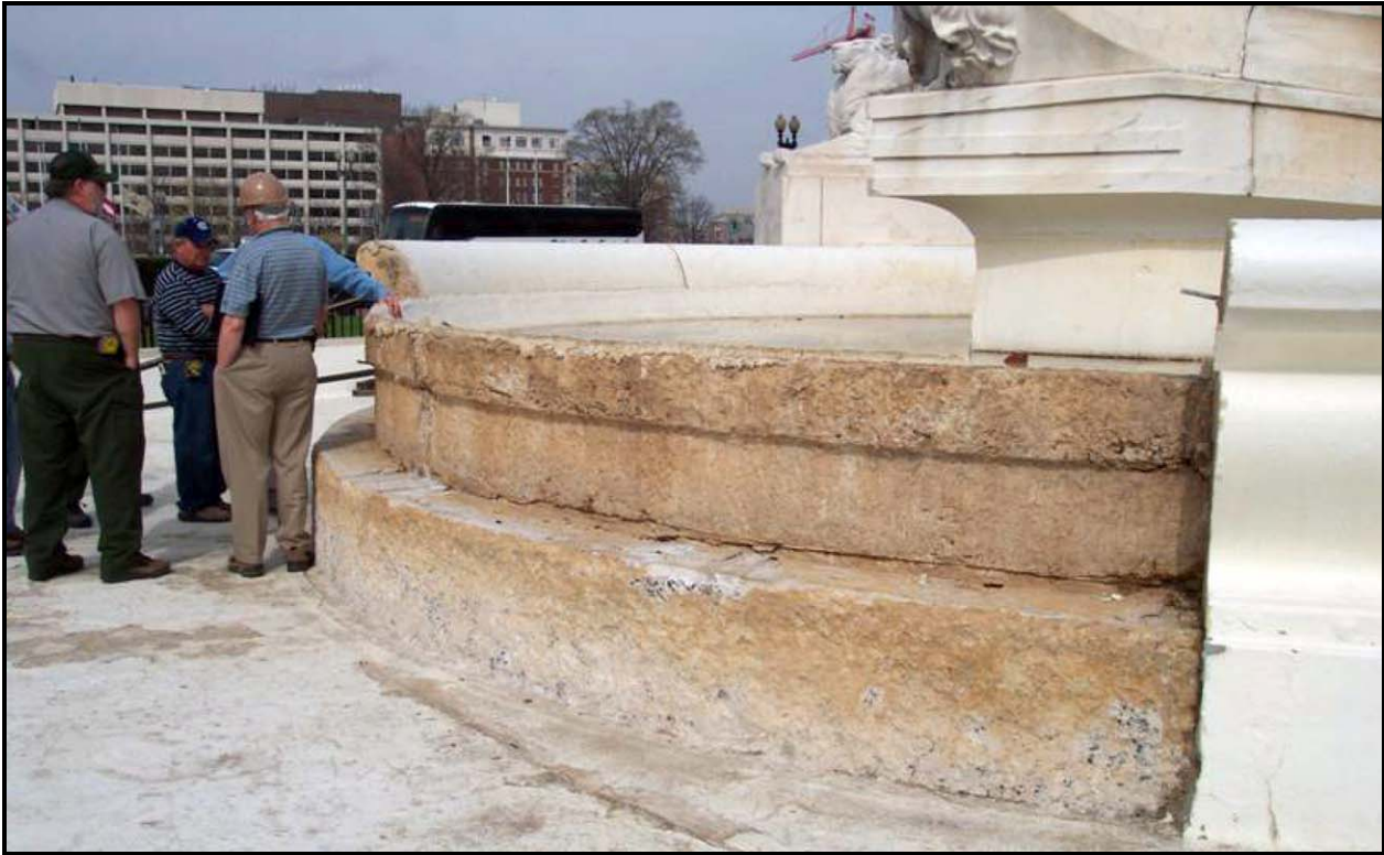
Figure 18. MISSING SKIRT STONES RESULTING FROM FAILURE OF THE UPPER BOWL RIM, COLUMBUS MEMORIAL FOUNTAIN, MARCH 2005
