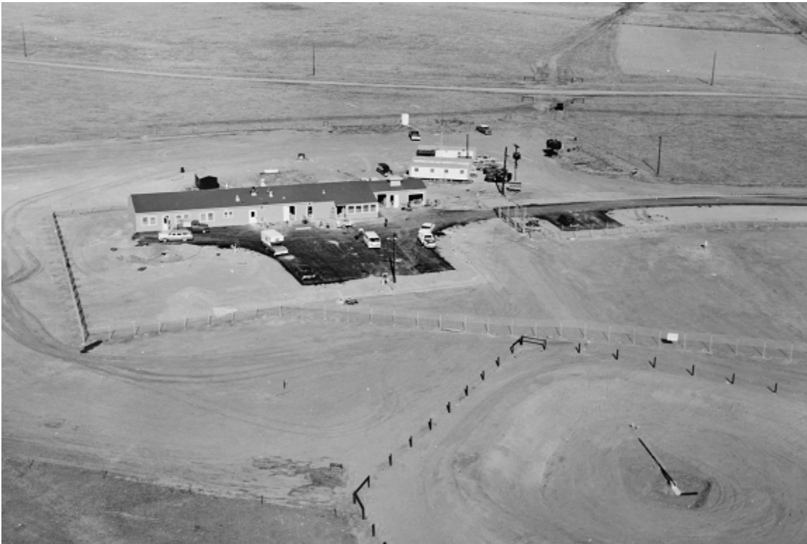
Figure 2- 4: Aerial oblique view of Delta-01 launch control facility under construction, parking area and approach road completed, sewage lagoon at lower right, ca. 1962
