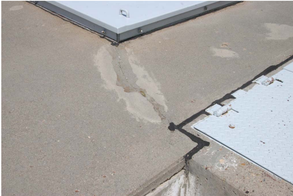
Figure 3- 75: Previously patched cracks at Delta-09 (source: FSE 010)
