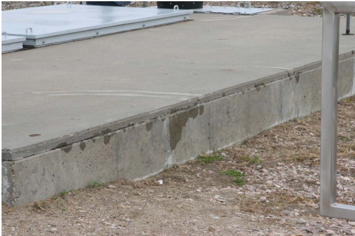
Figure 3- 76: Moisture migrating out from cracks at Delta-09 (source: FSE 051).
