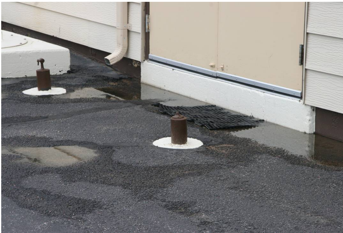
Figure 3- 46: Ponding at south elevation foundation wall (source: QEA 0008)
