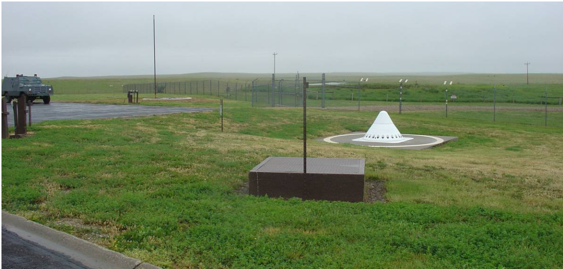
Figure 3- 12: Well cap (brown box) and Hardened Ultra High Frequency Antenna (white cone), facing southwest, June 2009 (source: QEA 3354)
