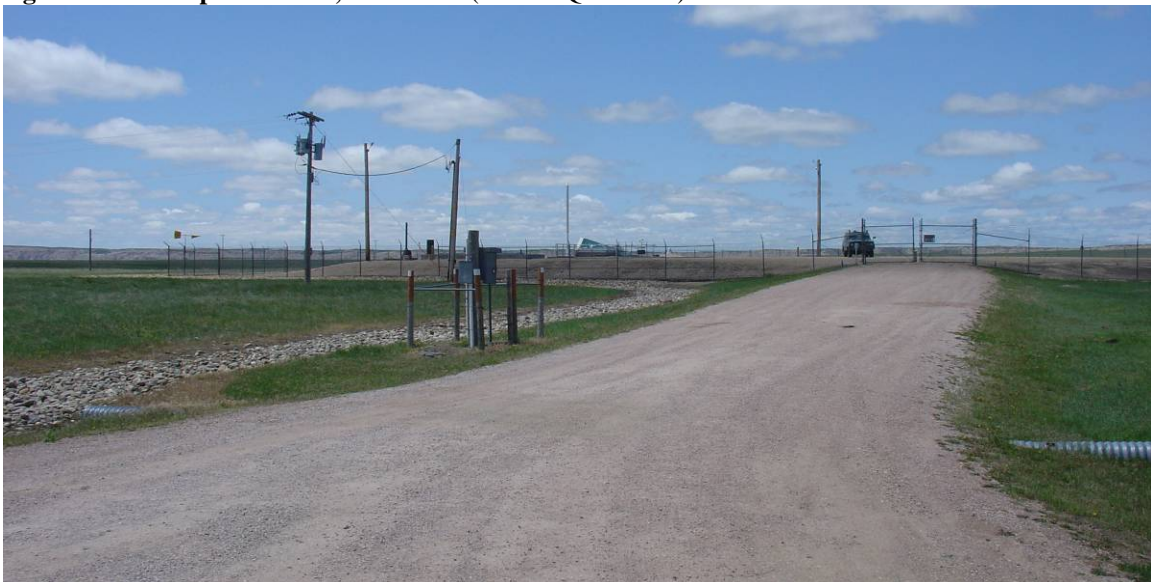
Figure 3- 41: Access drive at Delta-09, facing west, June 2009. Culvert under drive in foreground, cathodic protection device in middle, and gravel ditch to the left of the image. (source: QEA 3115)
