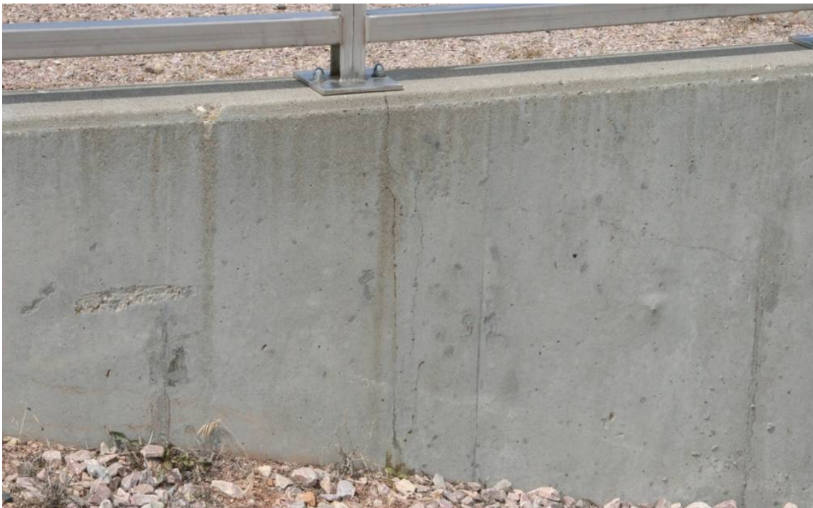
Figure 3- 79: Cracking in head walls at silo (source: FSE 040)
