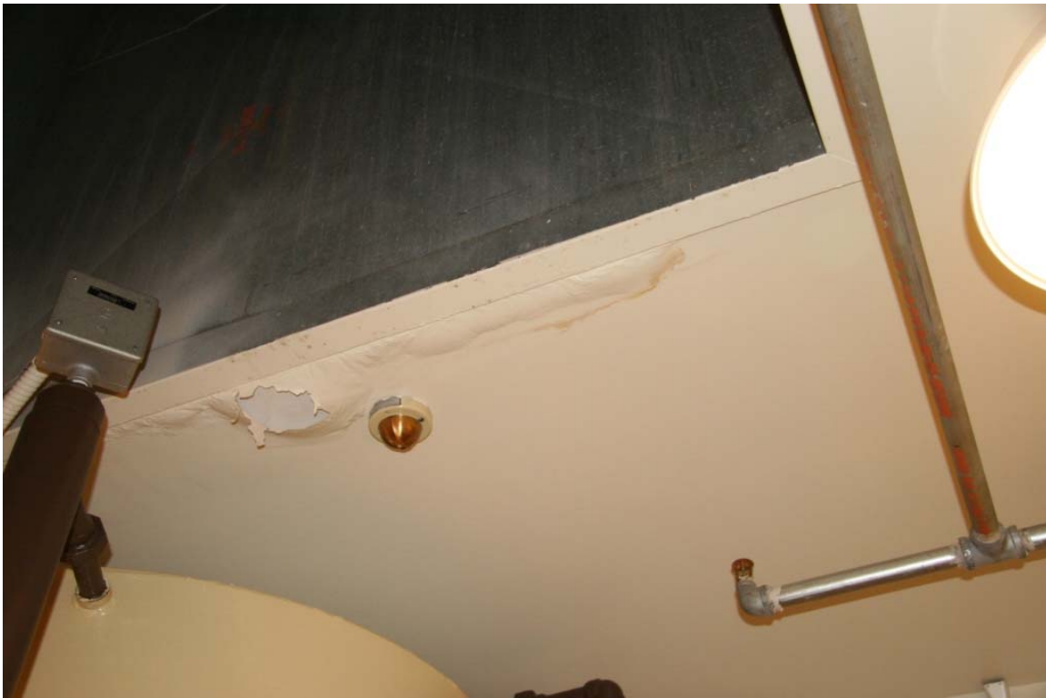
Figure 3- 73: Launch Control Support Building, flaking paint at Generator Room 105 (source: FSE 1056)
