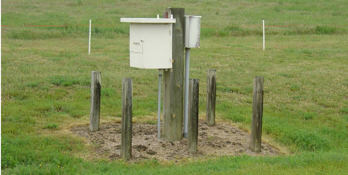
Figure 3- 13: Aboveground portion of the cathodic protection rectifier at Delta-01, facing northeast, June 2009 (source: QEA 3468)
