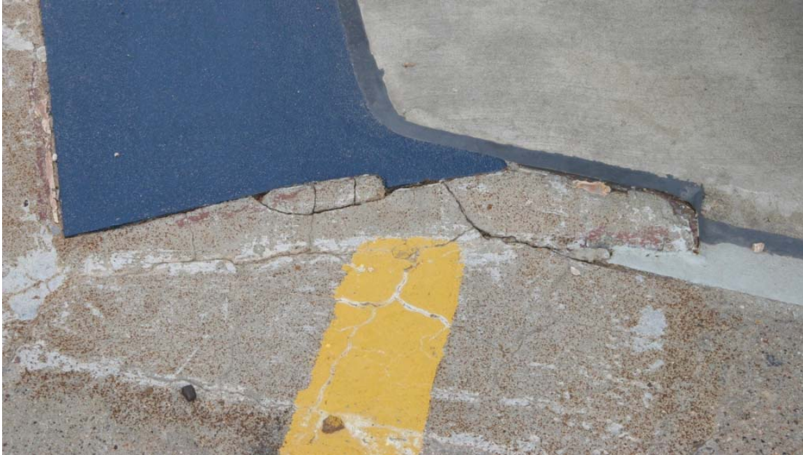
Figure 3- 78: Cracking of grout and concrete near silo metal plates (source: FSE 049)
