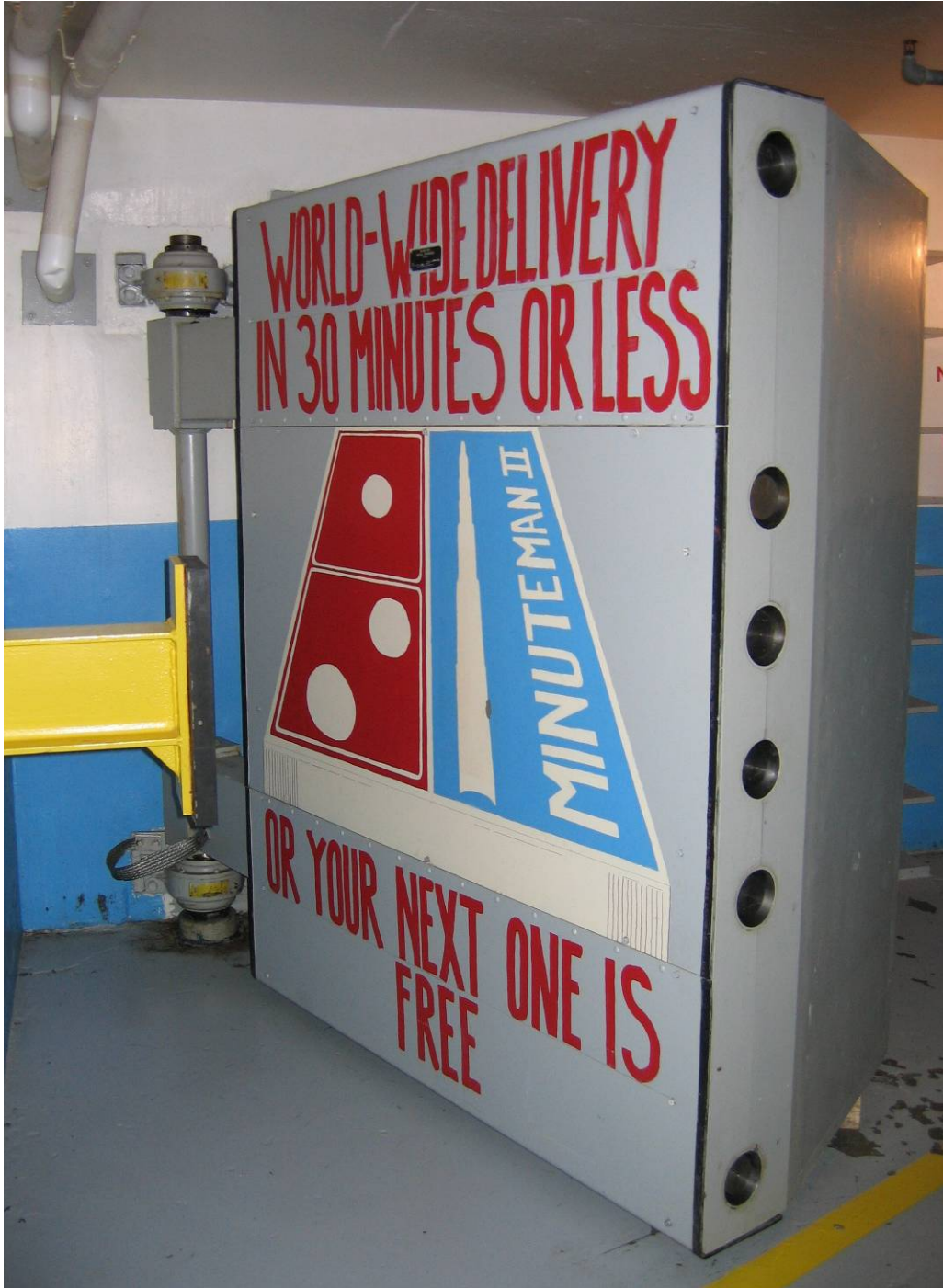
Figure 3- 62: LCC Vestibule, blast door (source: QEA 7015)
