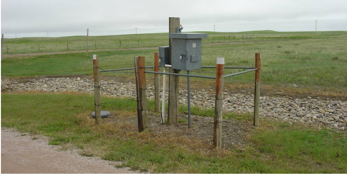
Figure 3- 35: Cathodic protection rectifier, facing southeast, June 2009 (source: QEA 3521)
