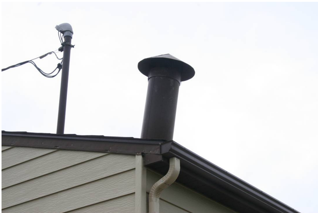
Figure 3- 68: Vehicle Heated Storage Building, gutters, downspouts, and vent (source: QEA 0026)
