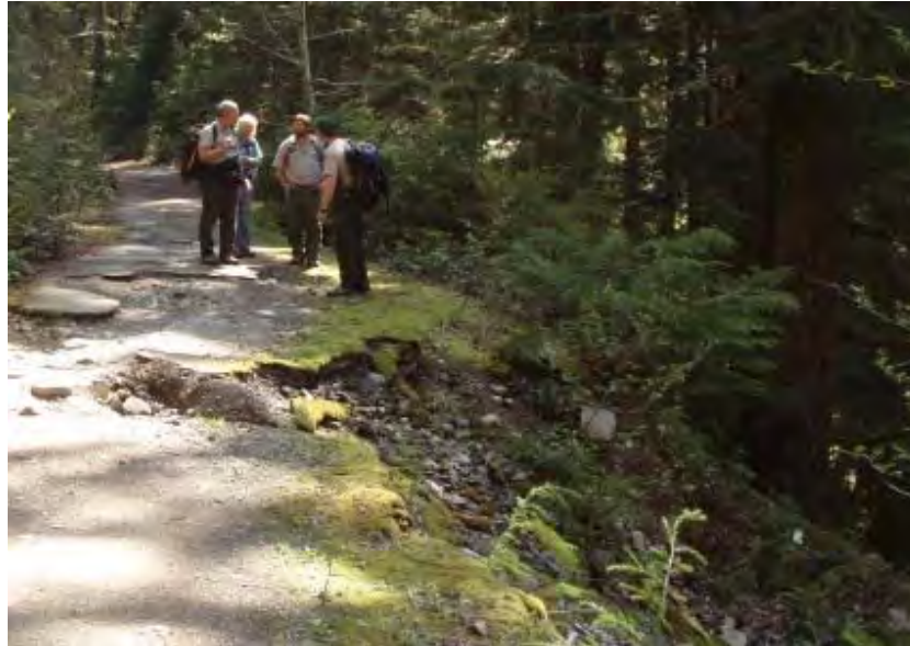
Photo 10: Deteriorating asphalt along the Boulder Creek trail.
