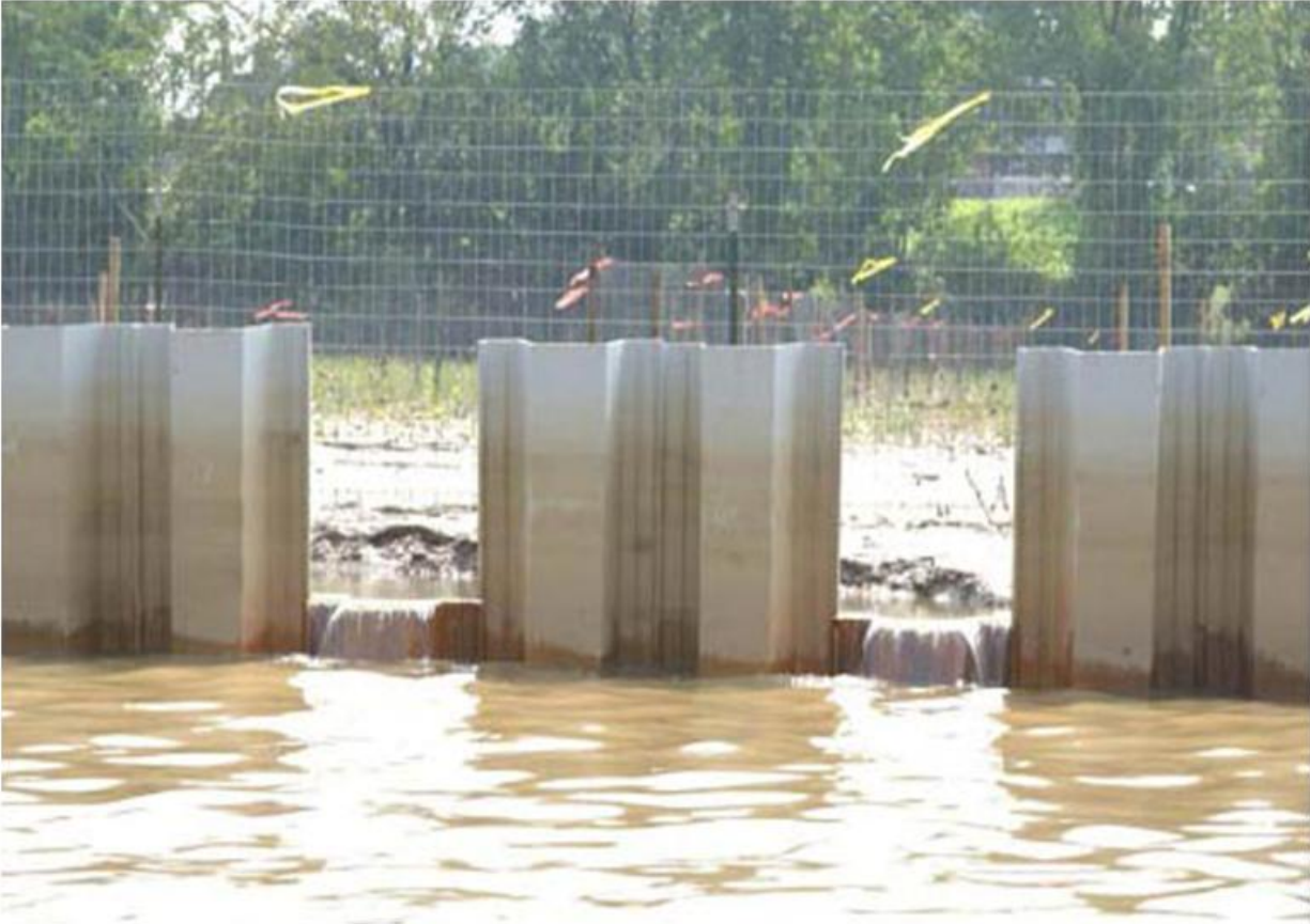
FIGURE 2-4. EXAMPLE OF SHEET PILING CONFIGURED TO ALLOW FOR INTERTIDAL EXCHANGE
