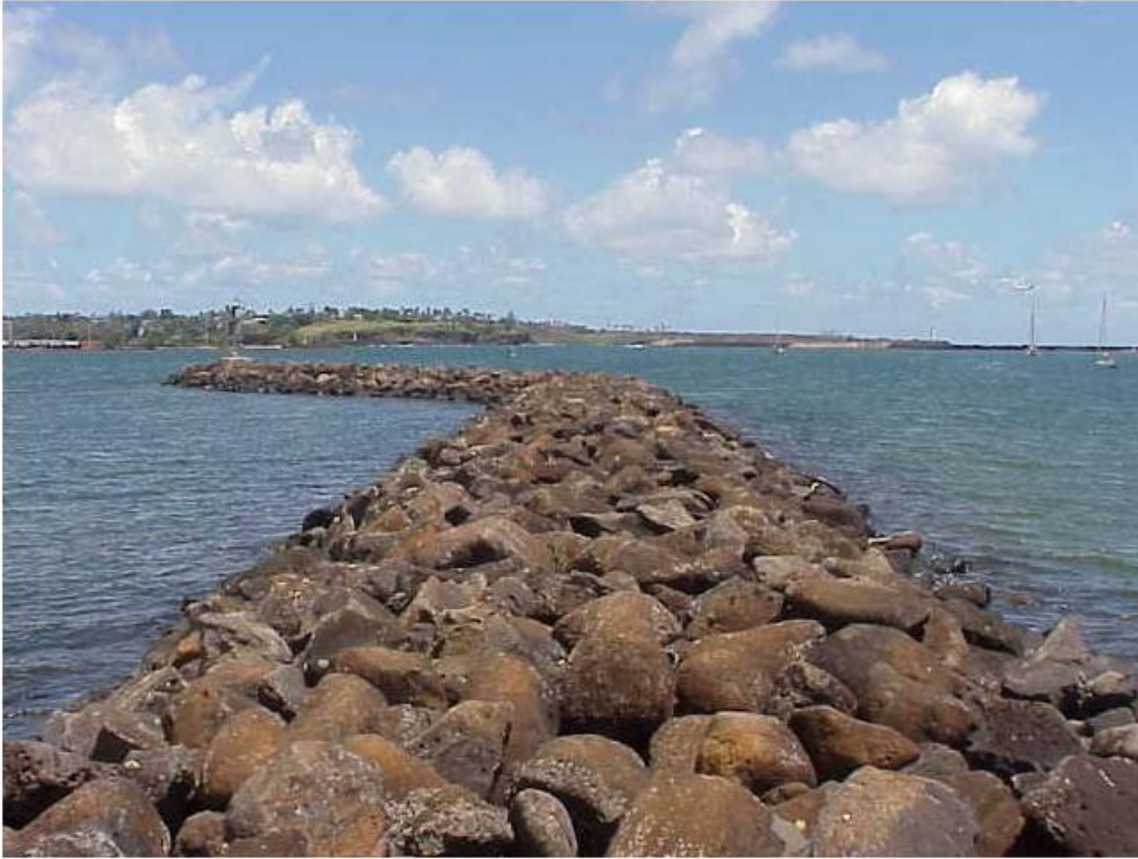
FIGURE 2-3. EXAMPLE OF A STONE BREAKWATER
