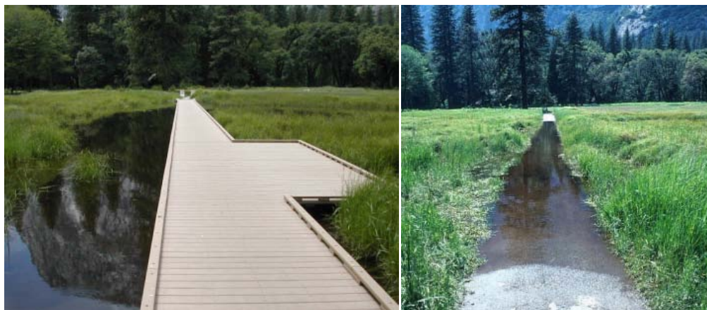
Figure 17: Trails through frequently inundated wet meadows, such as in cook's meadow pre-restoration (left), cause periperal vegetation trampling and soil compaction and make access difficult. A boardwalk installed in 2005 allows for visitor access into the meadow environment and protects the meadow soils and hydrology.
