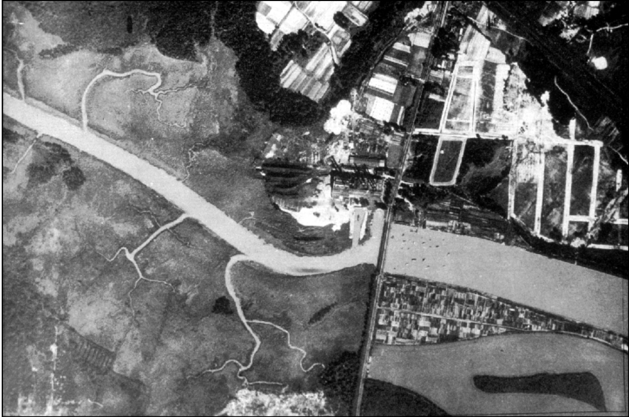
Benning Road Bridge 1927 across Anacostia River with dredged portion downstream (right side) and still intact freshwater tidal wetlands upstream (left side of photograph). Photo shows complete conversion of wetlands to fastland and tidal water below Benning Road (USGS 2006b).
