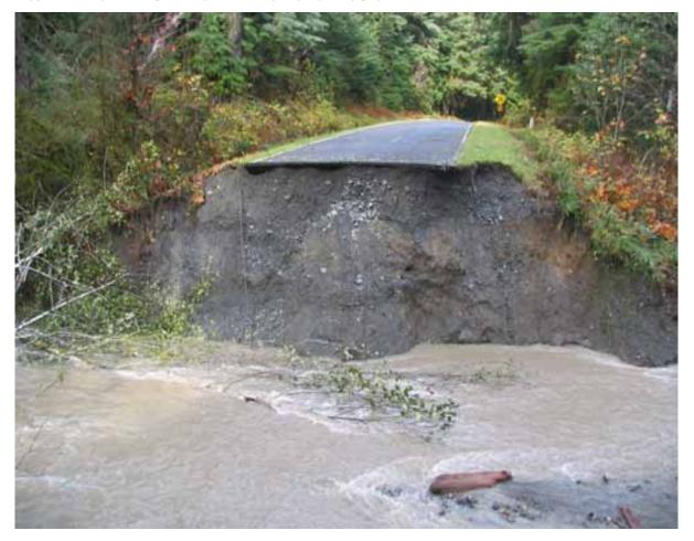
FIGURE 2. WEST TWIN CREEK ROAD DAMAGE FOLLOWING STORM
