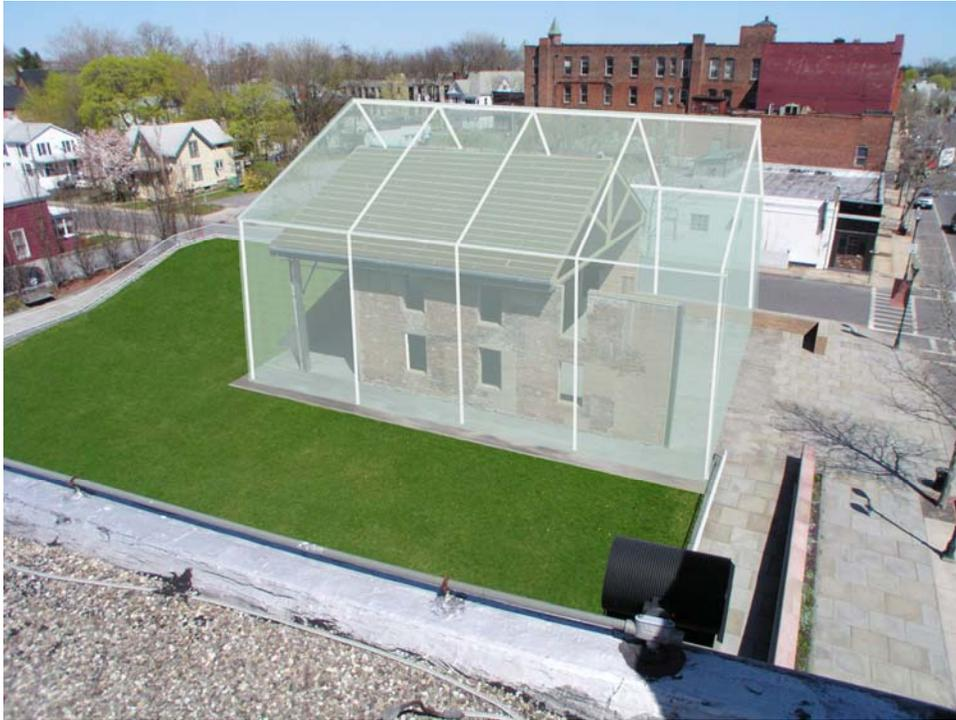
Figure 16: Alternative E - Enclose Chapel Remains in a New Structure
