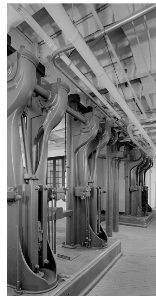
The pistons that ran the machinery of the Colt East Armory can still be seen in the lobby beneath the blue onion dome. Jet Lowe, Historic American Engineering Record , National Park Service.
