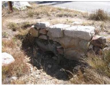
Partially blocked culvert.
