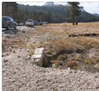
Fig. 1-17. Culvert set too low in meadow
