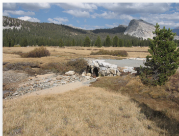
Fig. 1-26. Scour downstream of culvert on Unicorn Creek
