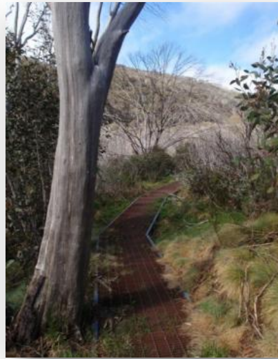
Figure – 3-6: Metal grate boardwalk in Australia
