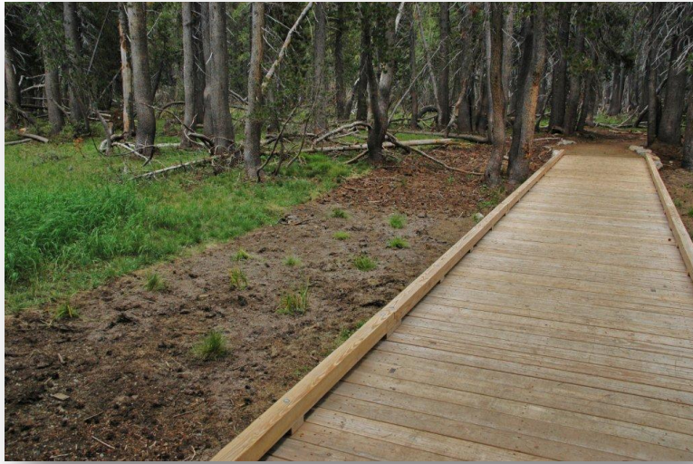
Figure 3-2: Newly installed TimberSIL® boardwalk at Tenaya Lake 2012
