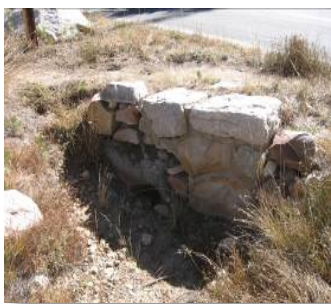
Fig. 1-16. Partially blocked culvert
