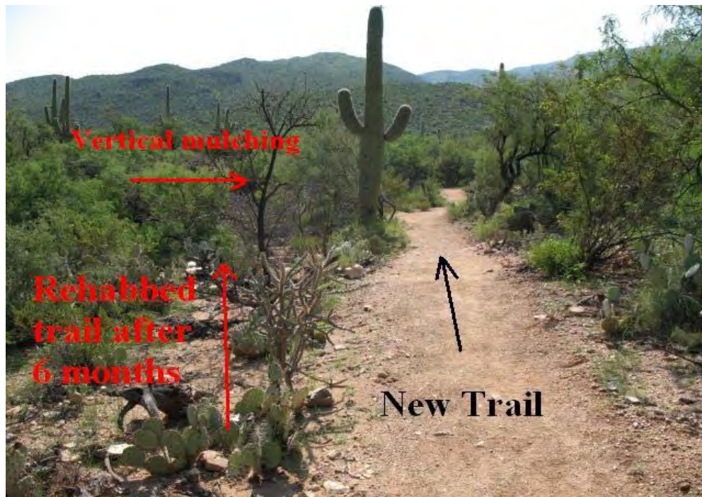
Rehabbed trail after 6 months; crew used fill material planting and vertical mulching on old trail
