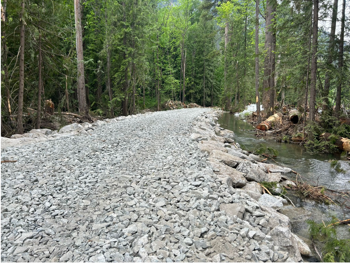
Figure 2. Existing NPS temporary road constructed in spring 2026 to provide emergency access to private property owners above washout on Company Creek Road, view west.
