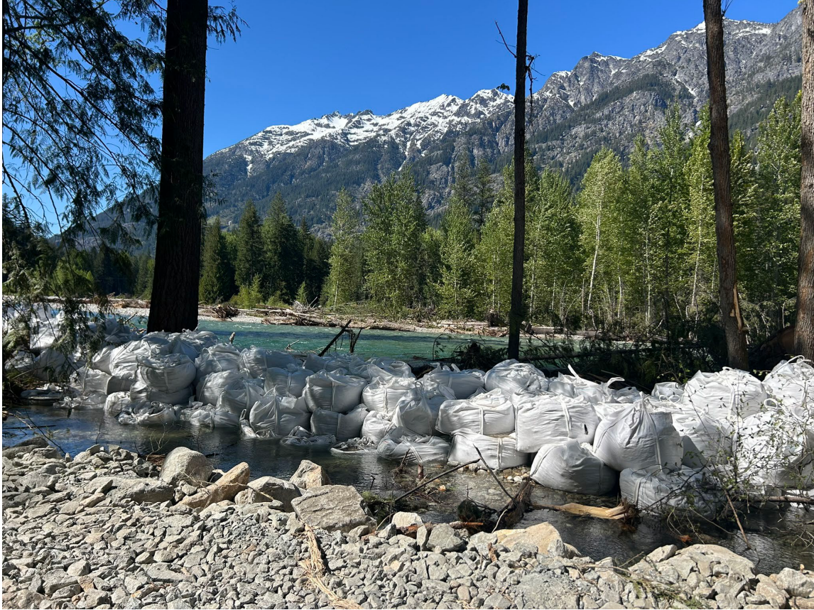
Figure 5. Existing temporary water barrier in front of NPS emergency road during the Stehekin River spring runoff that may be replaced with an improved barrier.
