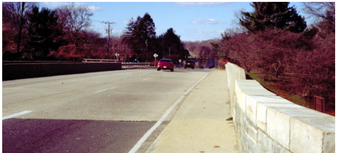
The existing sidewalk on the overpass is approximately 6 feet wide and 180 feet long. It is recommended that signage be provided at both ends of the sidewalk notifying users to cross in single file, and to dismount bicycles and walk them across.
