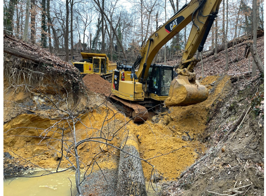
Access via Stream Channel
