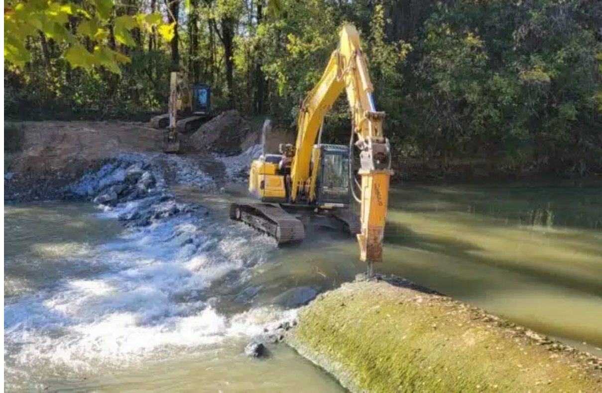
Representative image of excavator removing a shallow concrete dam.
