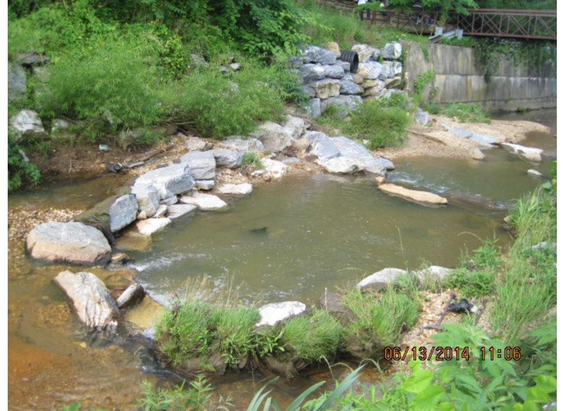
Sewer Infrastructure in Stream- After
