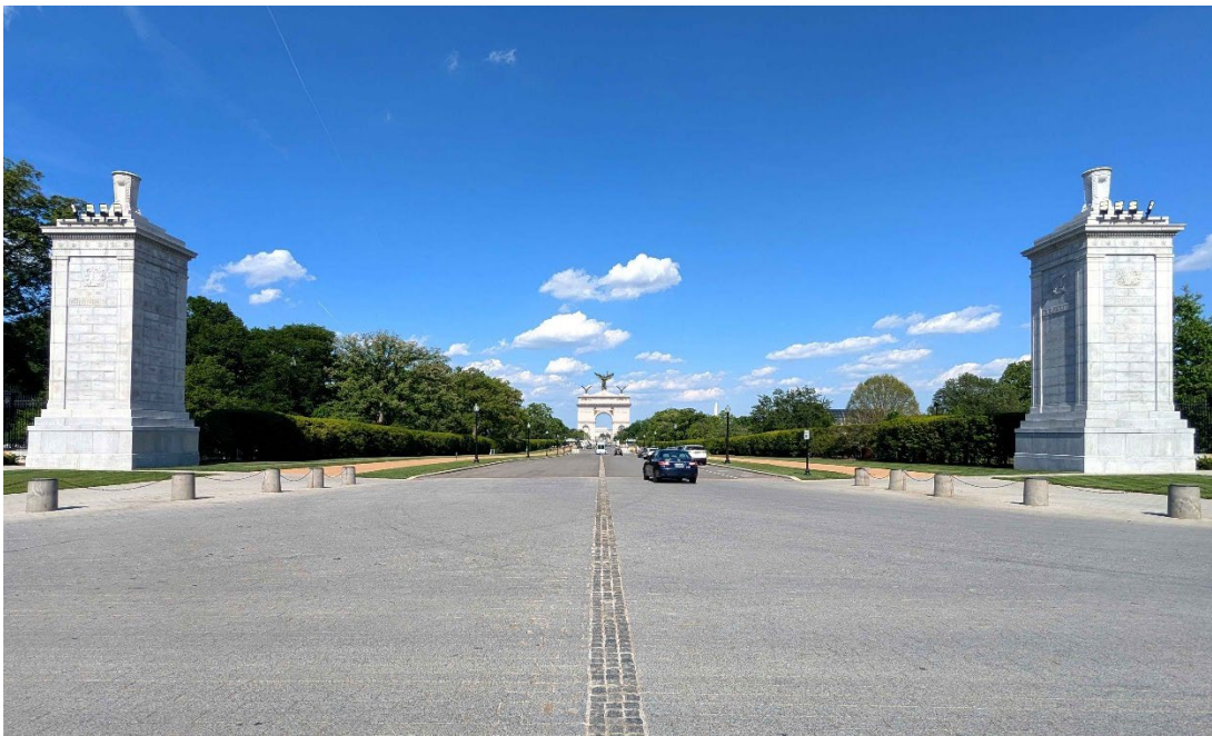
Image 11. View from the Arlington Hemicycle toward the Lincoln Memorial with the proposed Triumphal Arch. ©Harrison Design
