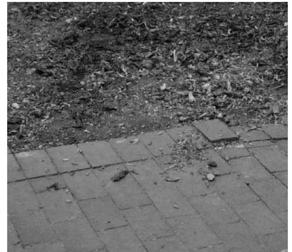
Site Visit Photos, 2026
