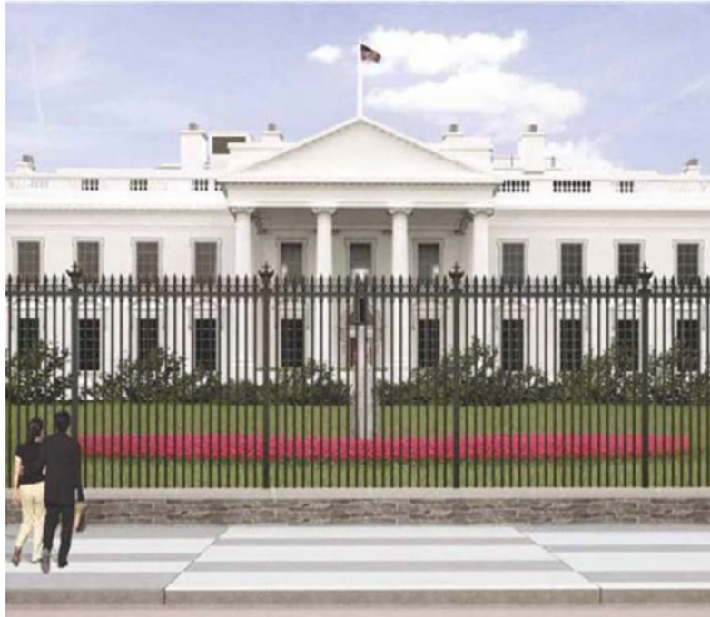
White House Fence
