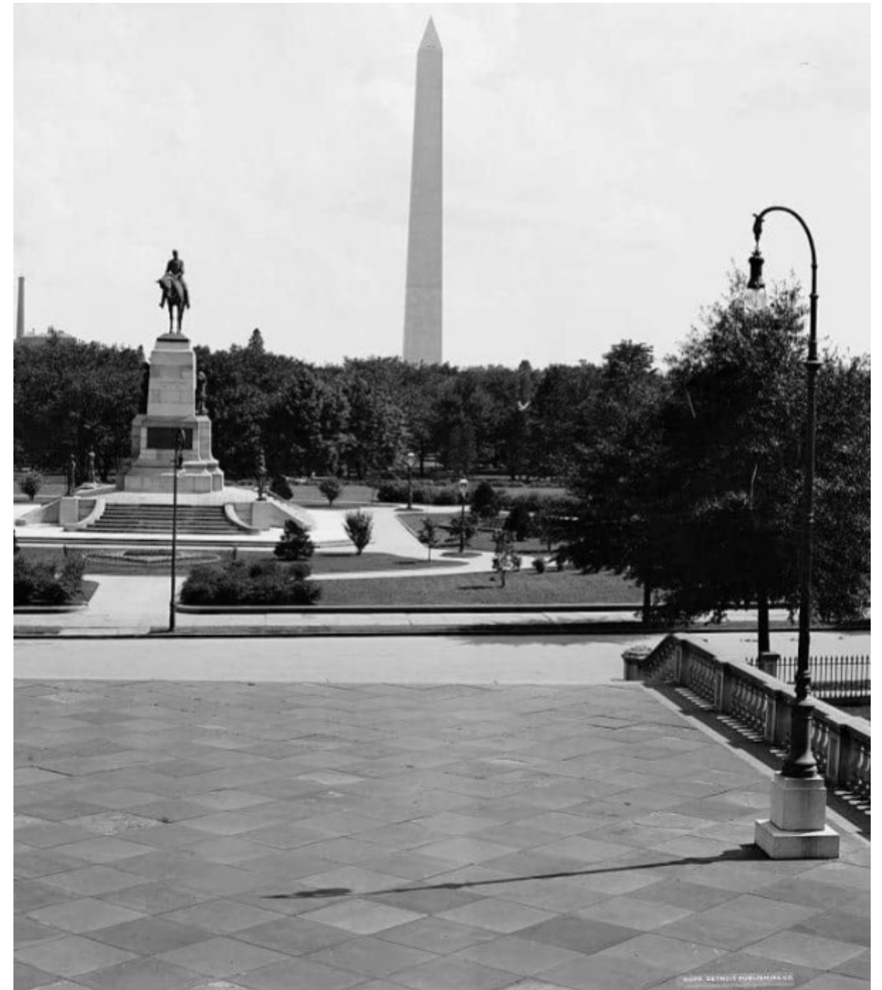
1903: Original sidewalks installed; View south
