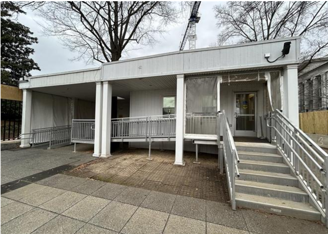
East Executive Avenue, existing visitor screening trailer, looking north, Treasury Department is on the far right.
